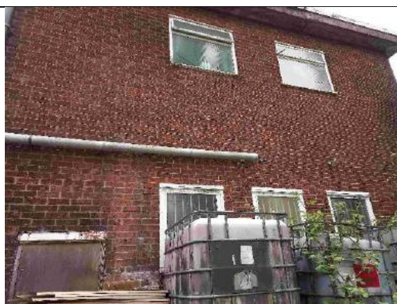
Photograph 20: Eastern elevation of B4
