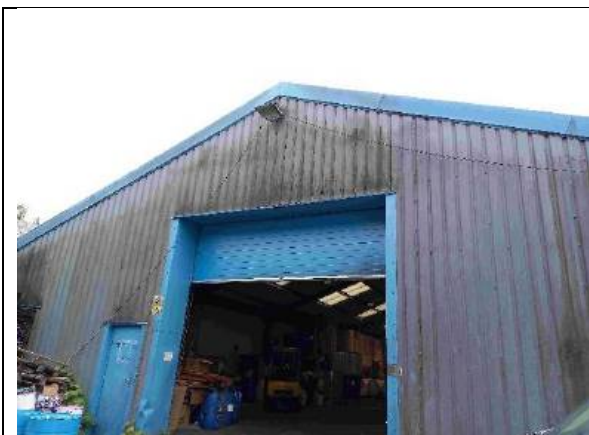
Photograph 17: Western elevation of B3
