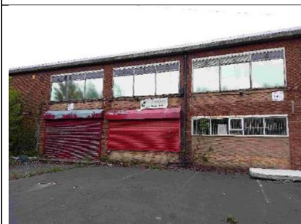
Photograph 19: Southern elevation of B4
