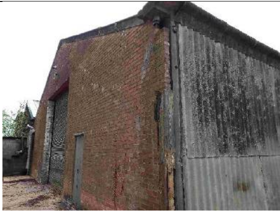
Photograph 13: Eastern and northern elevation of building B2
