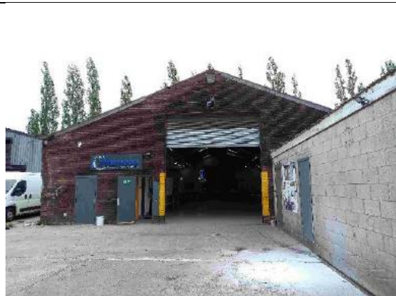
Photograph 16: Western elevation of B2 with single storey extension
