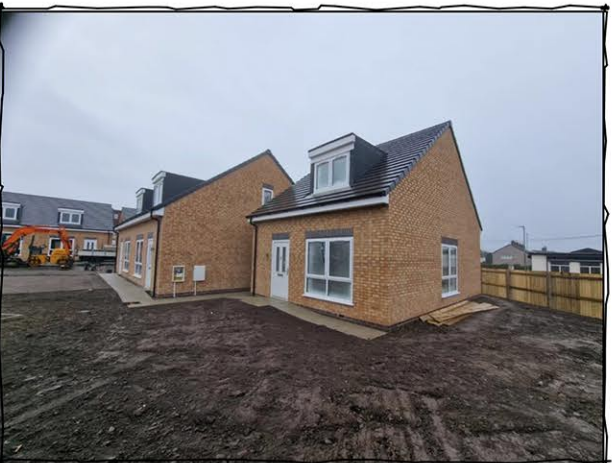
Photo 4 - Corner View of Unit 9
