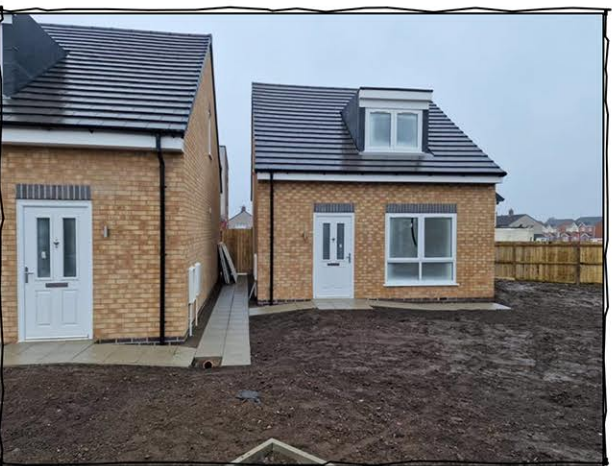
Photo 3 - Front View of Unit 8 & 9
