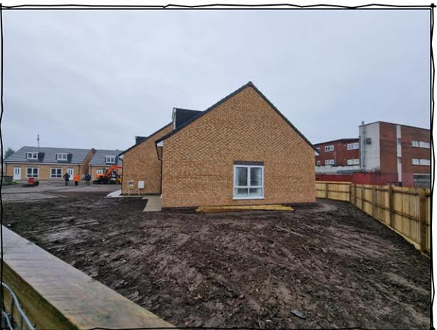
Photo 2 - End Gable of Unit 9
