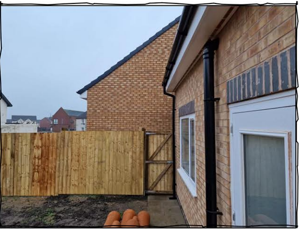
Photo 1 - Side View from Unit 8
