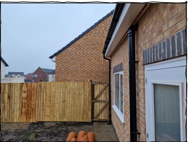
Photo 1 - Side View from Unit 8
