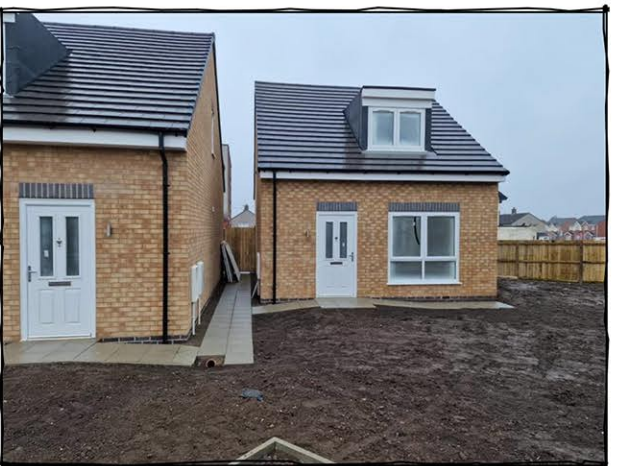
Photo 3 - Front View of Unit 8 & 9
