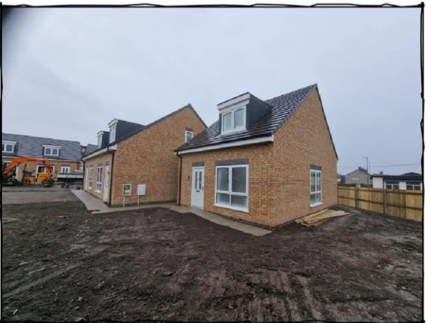
Photo 4 - Corner View of Unit 9
