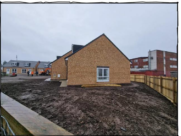
Photo 2 - End Gable of Unit 9
