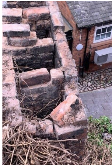
Part way through works
