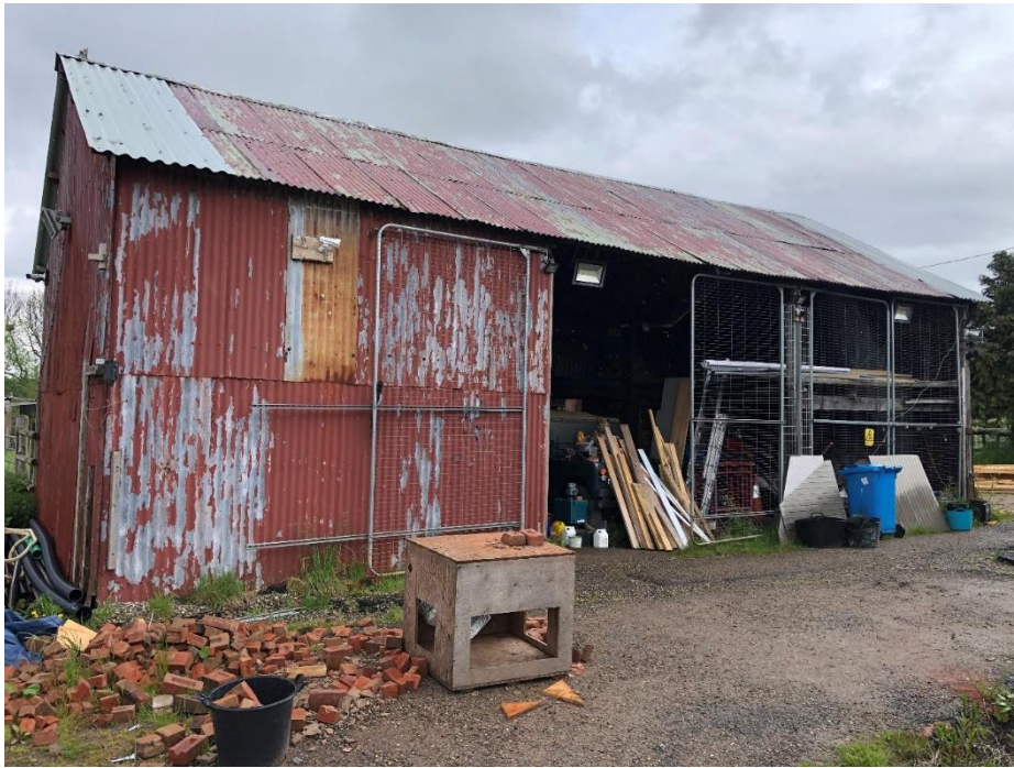
Figure 3 – Existing Barn, South Elevation.
