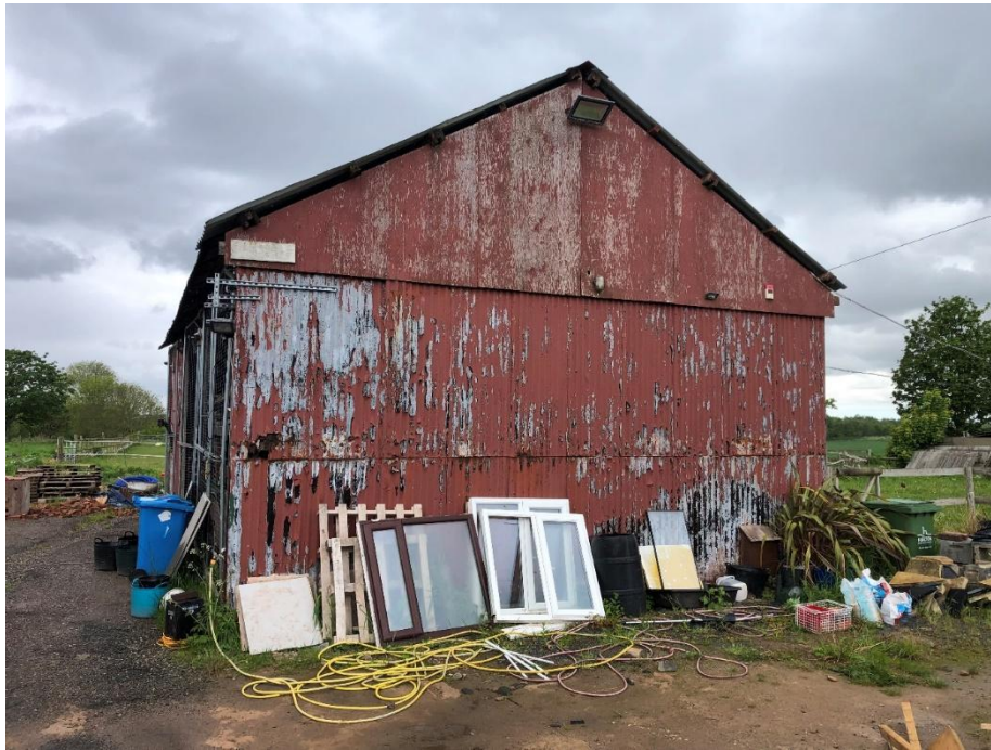
Figure 1 – Existing Barn, East Elevation.
