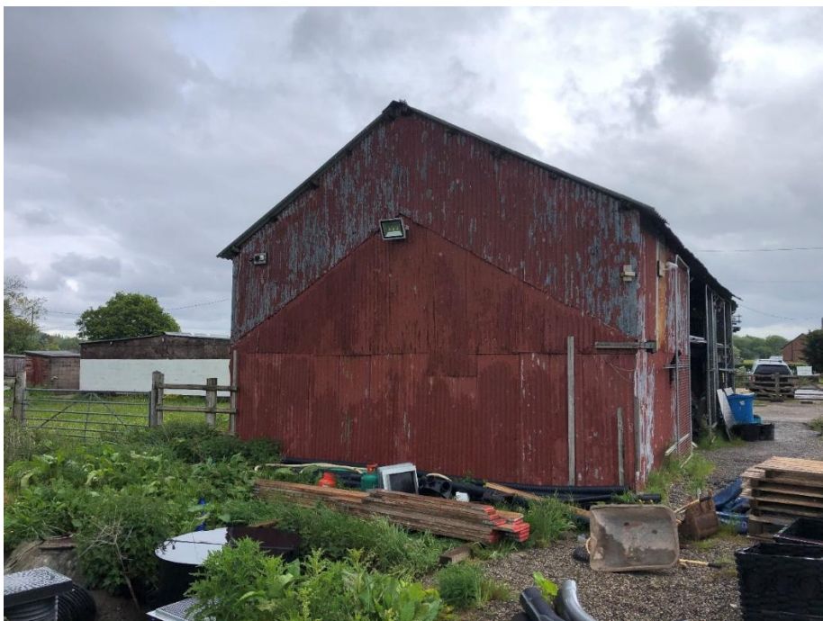
Figure 2 – Existing Barn, West Elevation.
