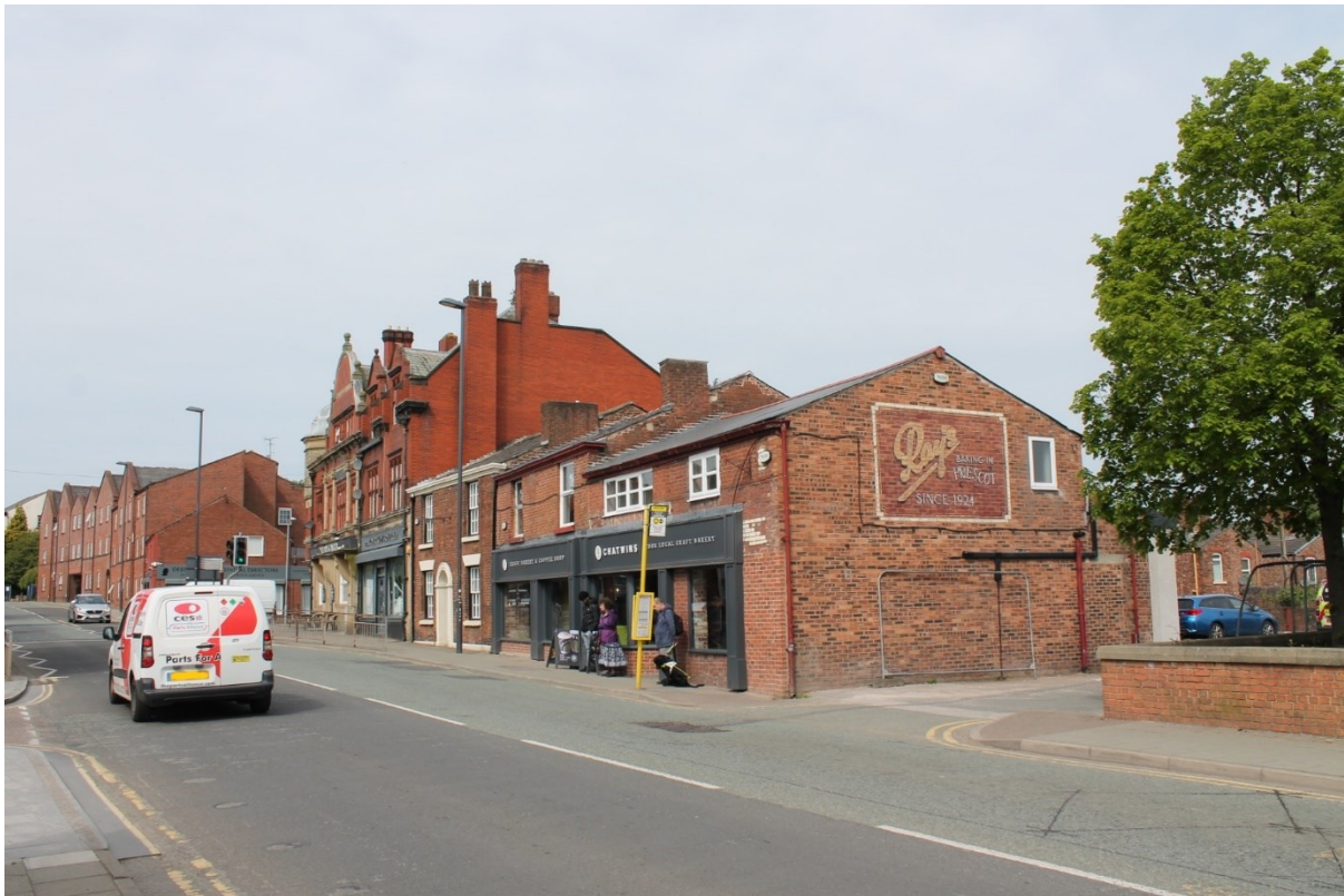
Figure 2.3: Application property and adjoining buildings
