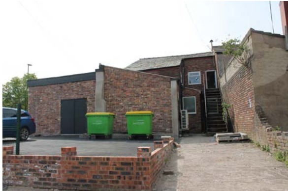
6. View of rear of bakery and entrance to first floor flat
