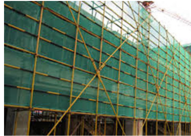
Figure 13. Debris netting
