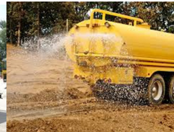
Figure 16. Dust Suppression
