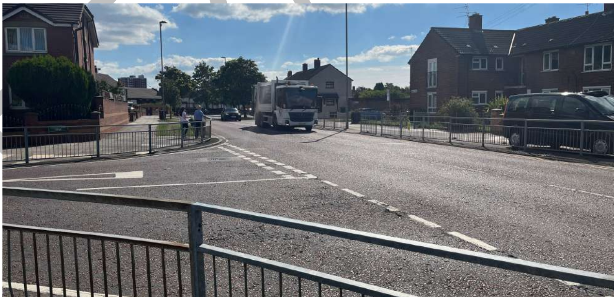
Photograph 2.8 : Bewley Drive / Cherryfield Drive
