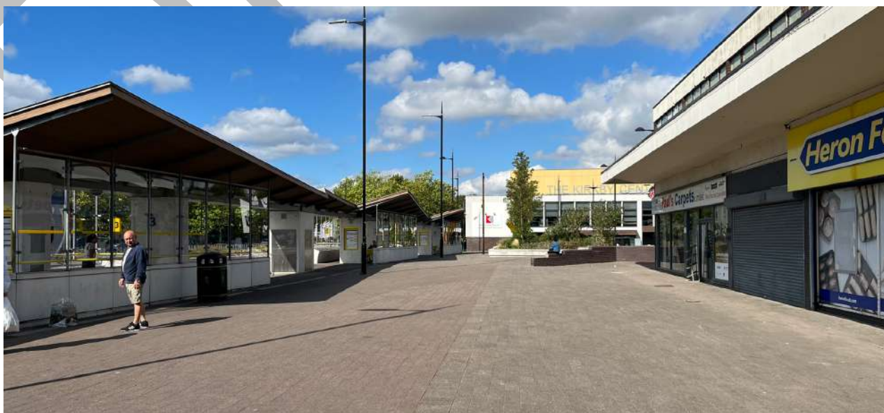
Photograph 3.1 : Kirkby Bus Station
