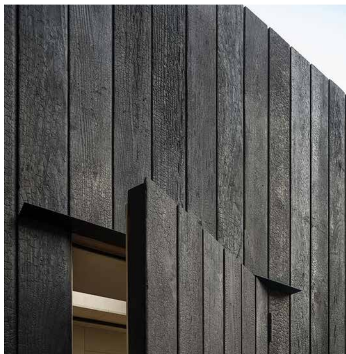
Black Timber Cladding
