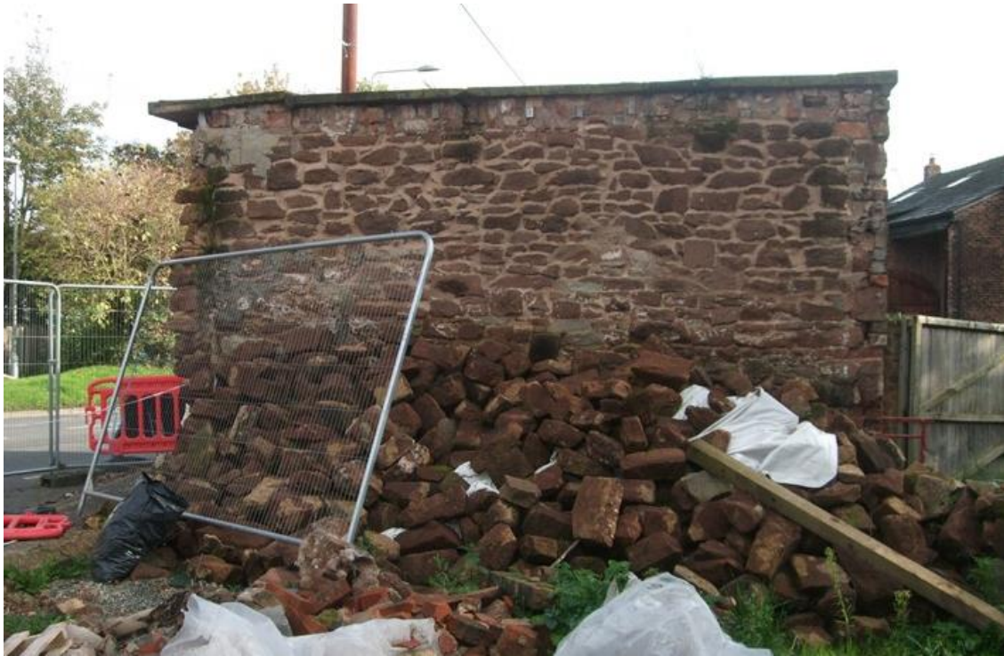
Figure 3: Still-standing portion of original wall, perpendicular to section requiring reconstruction (at left)
