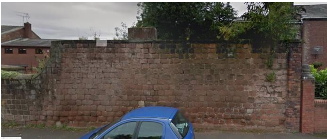
Figure 4: Original appearance of front elevation of currently dismantled boundary wall (image: Google Streetview)
