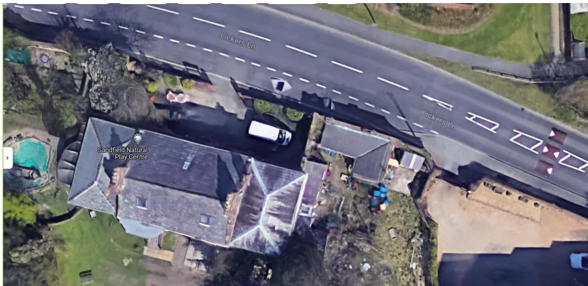
Figure 5: Aerial photograph of Sandfield House and former outdoor store to the immediate NE, prior to its removal (image: Google Maps)
