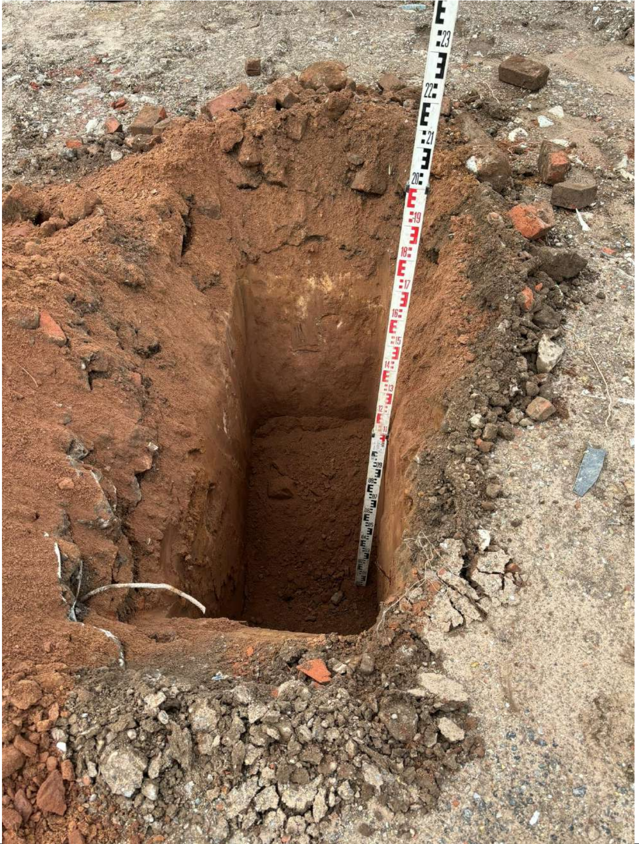
Plate 10: TP10 showing southern face and the depth of the excavation
