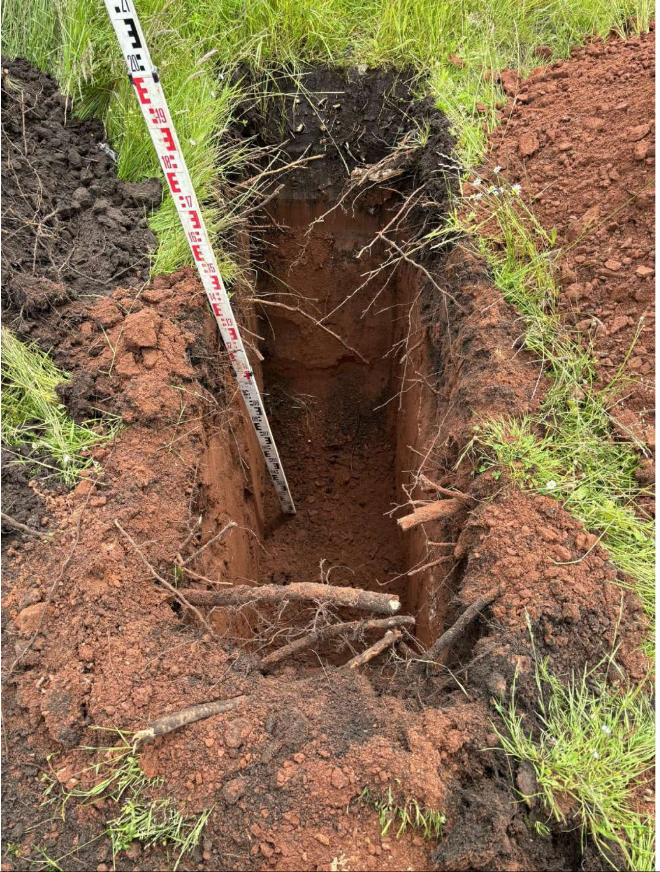
Plate 2: TP02 showing the southern face and base of excavation
