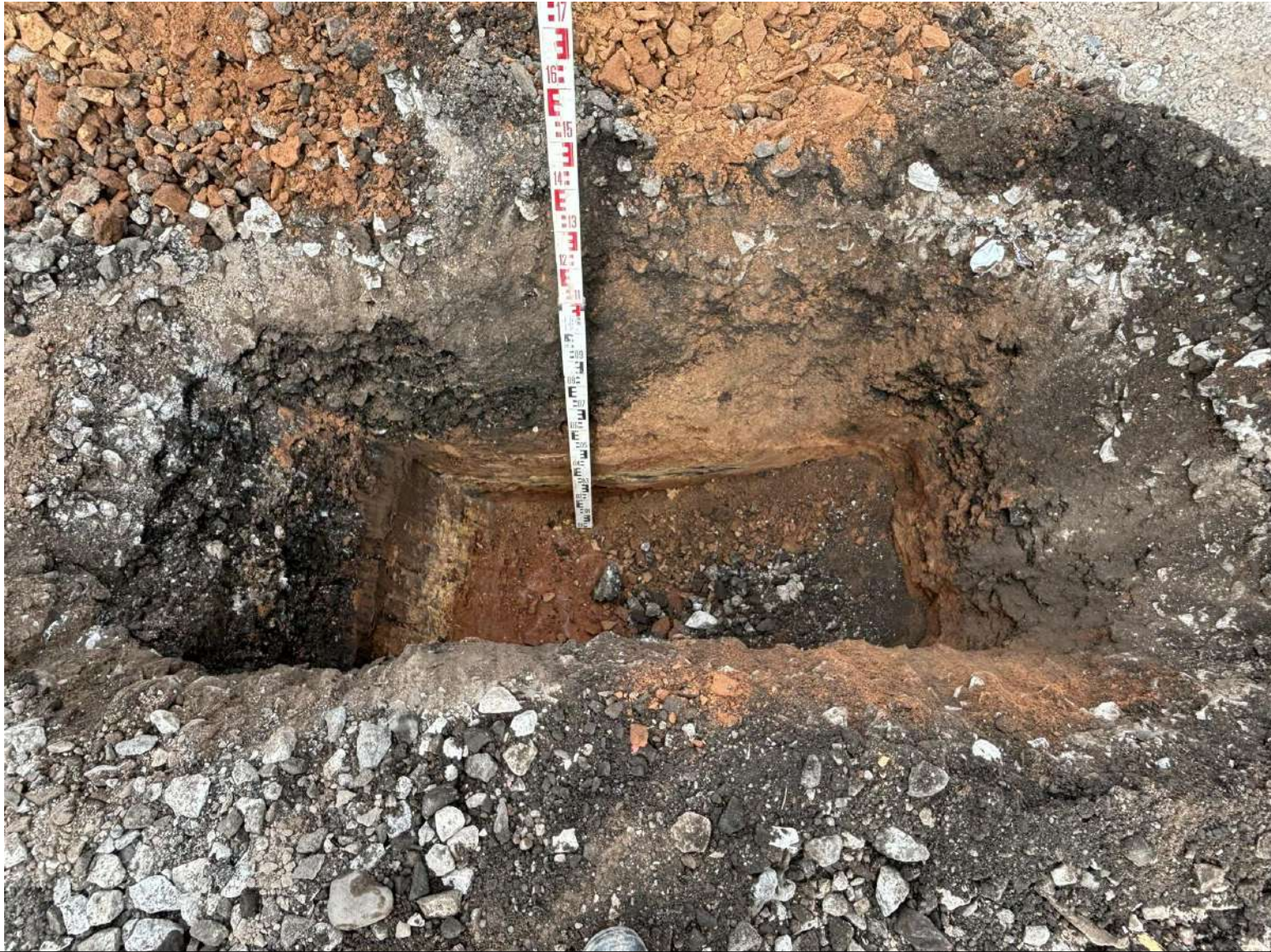
Plate 18: TP17 showing the base of the excavation and side walls
