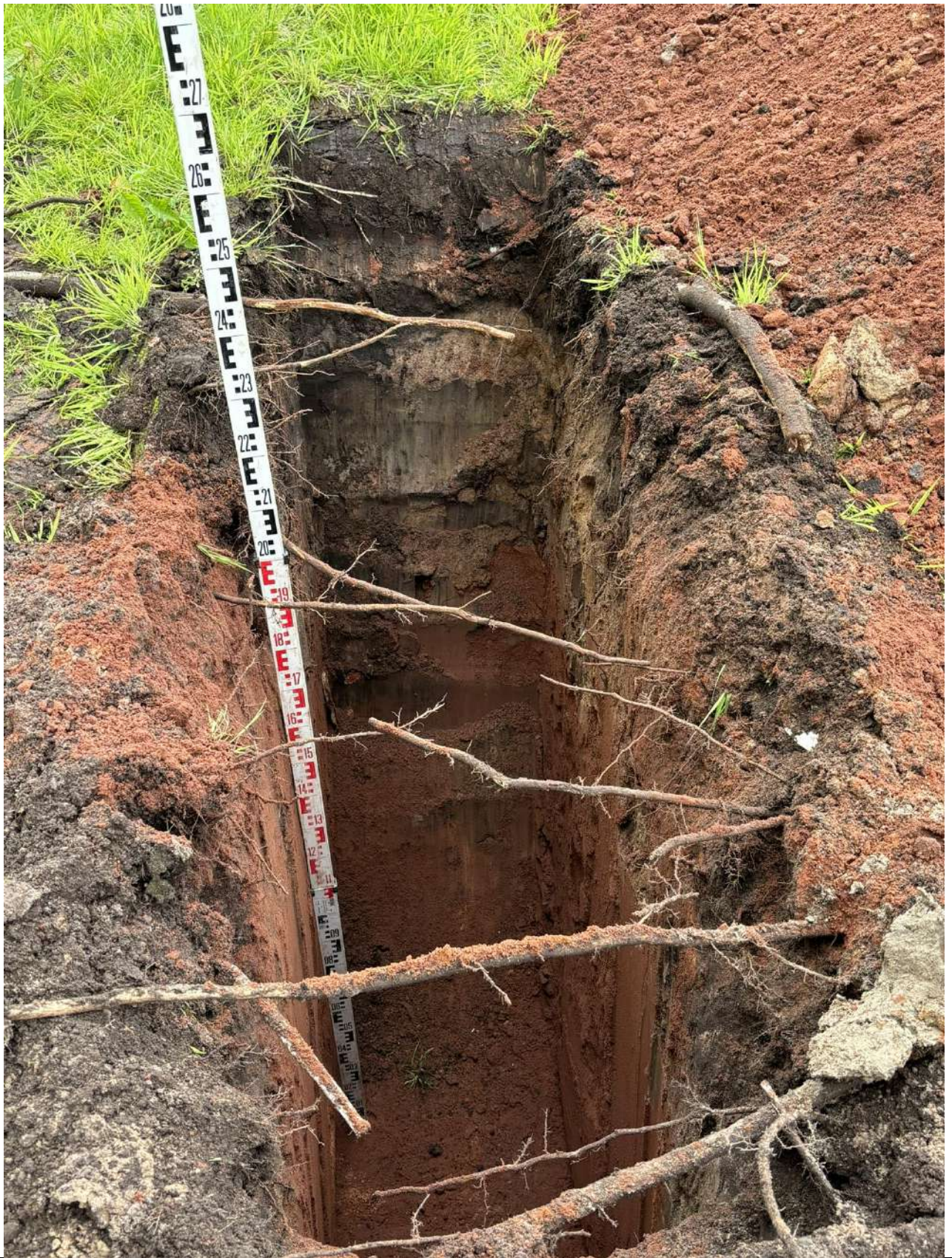
Plate 6: TP06 showing depth of excavation and roots encountered during the excavation
