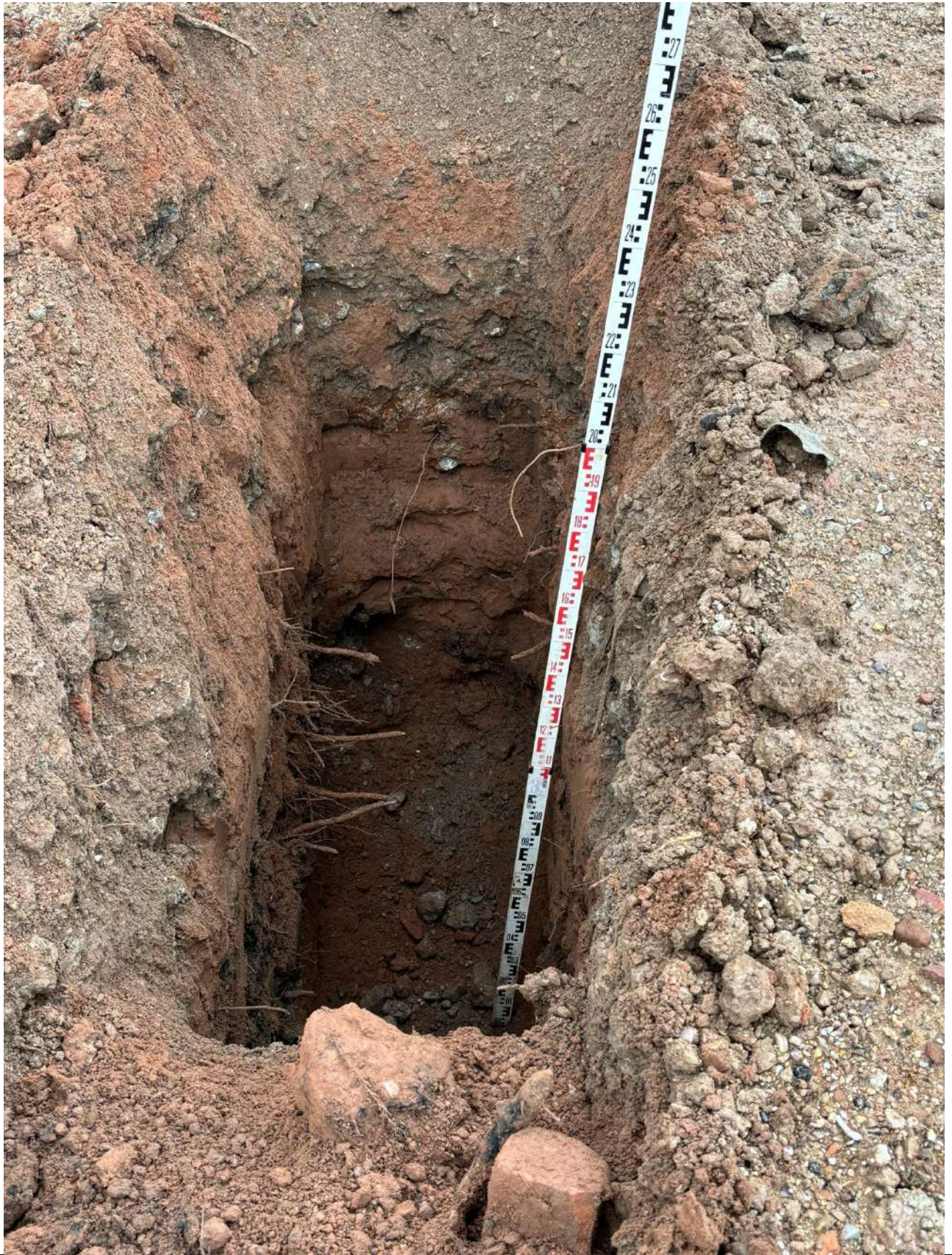
Plate 4: TP04 showing the depth of the excavation and stratigraphy
