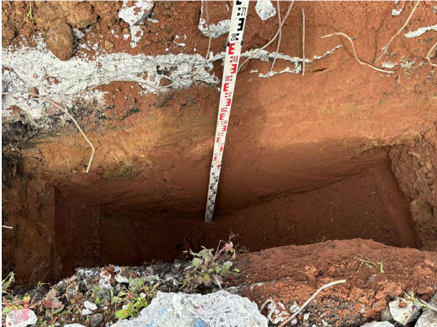
Plate 1: TP01 showing the base of the excavation and side wall
