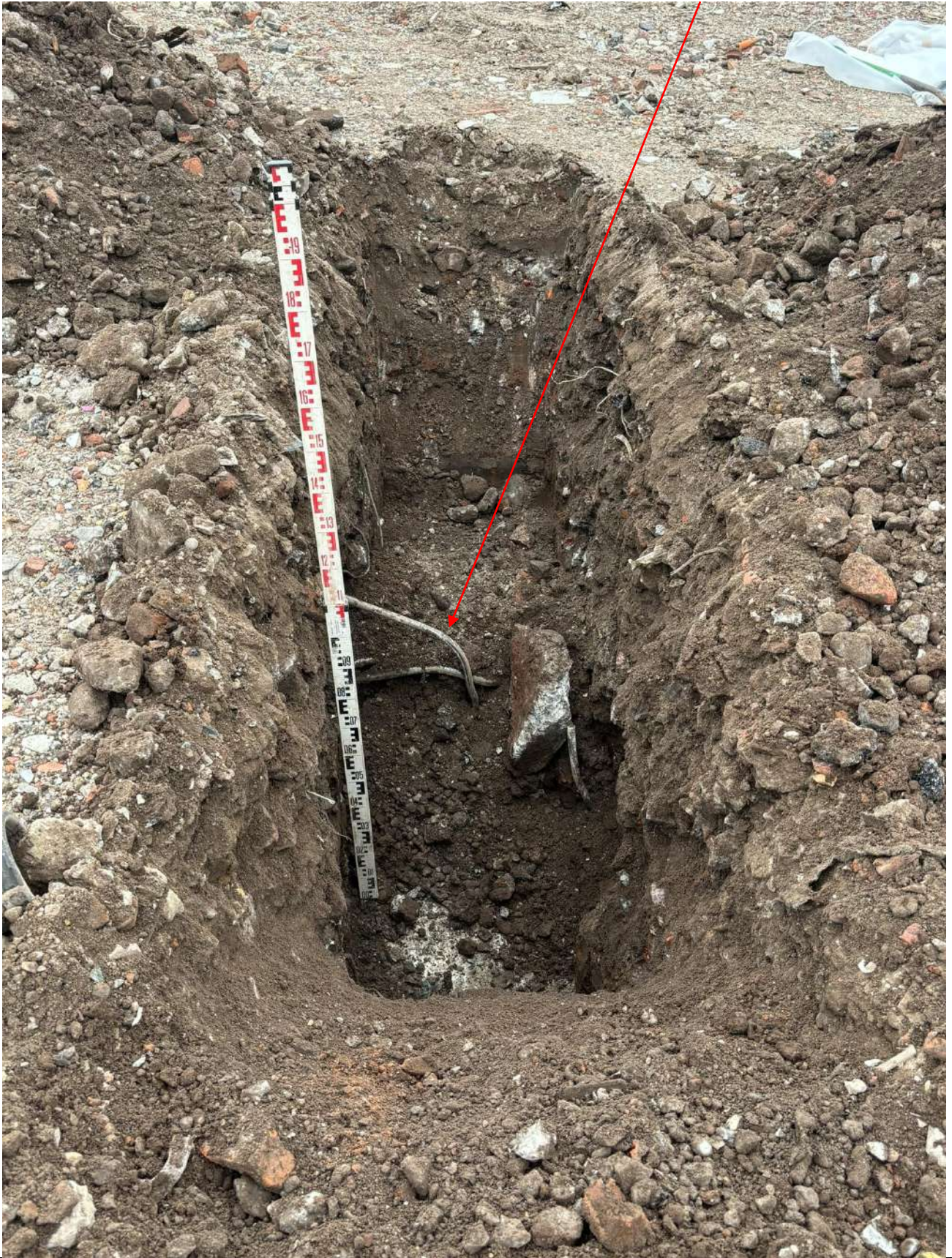
Plate 17: TP16 showing the base of the excavation and metal obstructions found
