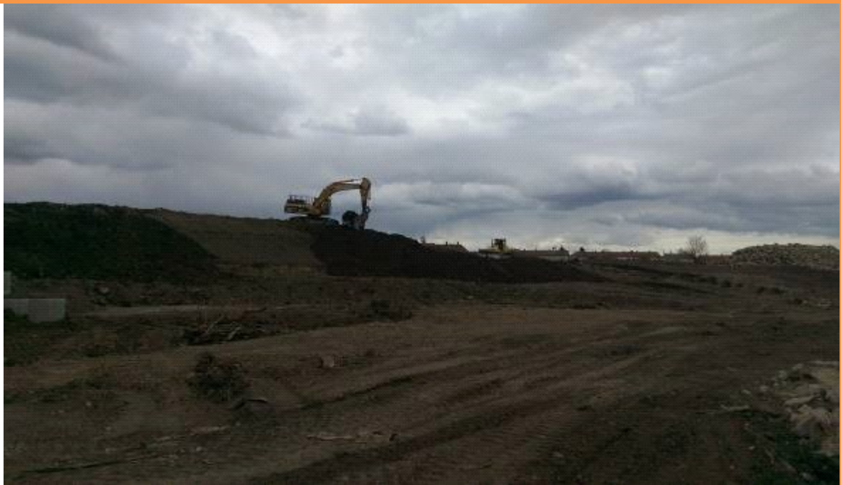
PLATE 21 – TURNOVER OF EMBANKMENT TO REDUCE THE SITE INTO ONE PLATEAUX
