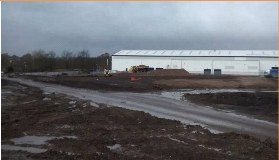
PLATE 15 – LOWER PARCEL C TURNOVER COMPLETE WITH SOILS BEING IMPORTED TO RAISE PARCEL
