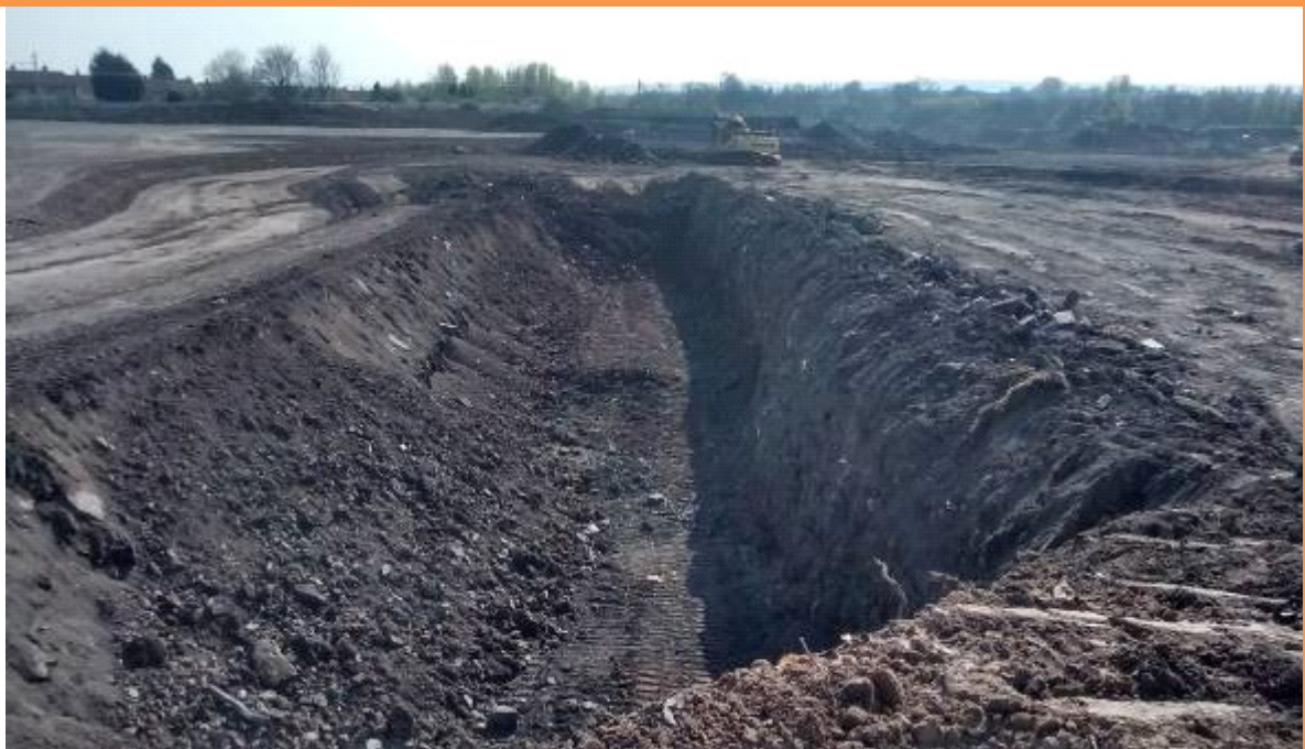
PLATE 18 – PARCEL C SOUTHERN BOUNDARY TURNOVER IN PROGRESS ADJACENT TO CONSTRUCTED SPINE ROAD
