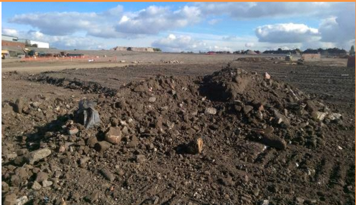
PLATE 24 – PARCEL C IN DISTANCE WITH REMEDIATION COMPLETE TO FORMATION LEVEL
