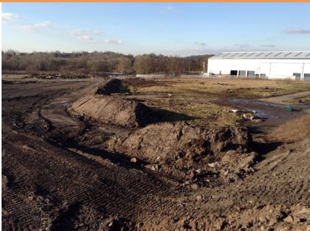
PLATE 2 – REMOVAL OF VEGETATION STRIP IN PROGRESS
