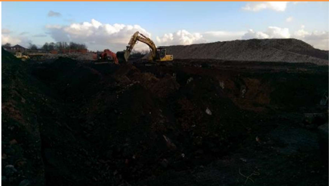
PLATE 6 – TURNOVER AND REMOVAL OF RELIC STRUCTURES
