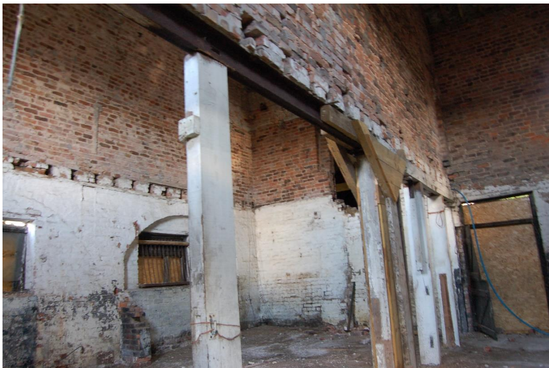
iii. Interior main barn (F8) (showing bays and arches in east facing elevation)
