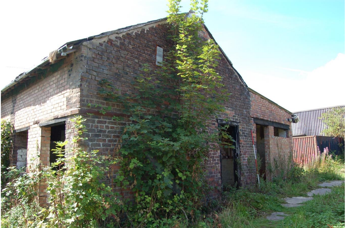
15. East facing elevation of storage barn
