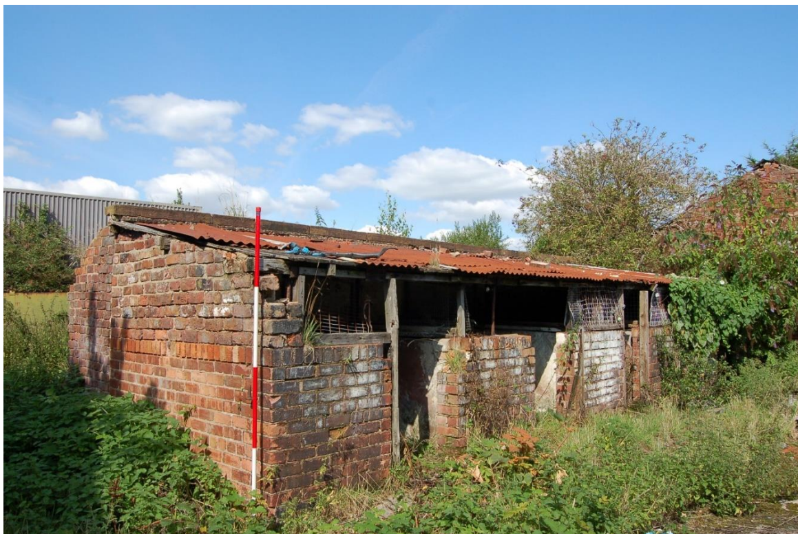
12. South and west facing elevations of pigsty
