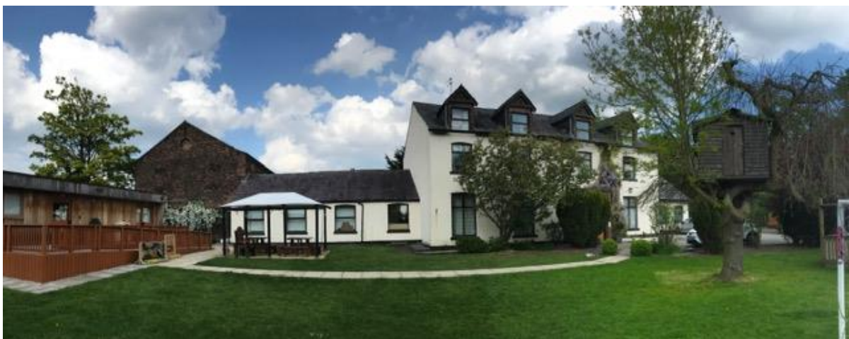
xiii. Main barn, west facing elevation (F8) with former farmhouse and attached barn (B1), both now within the school grounds
