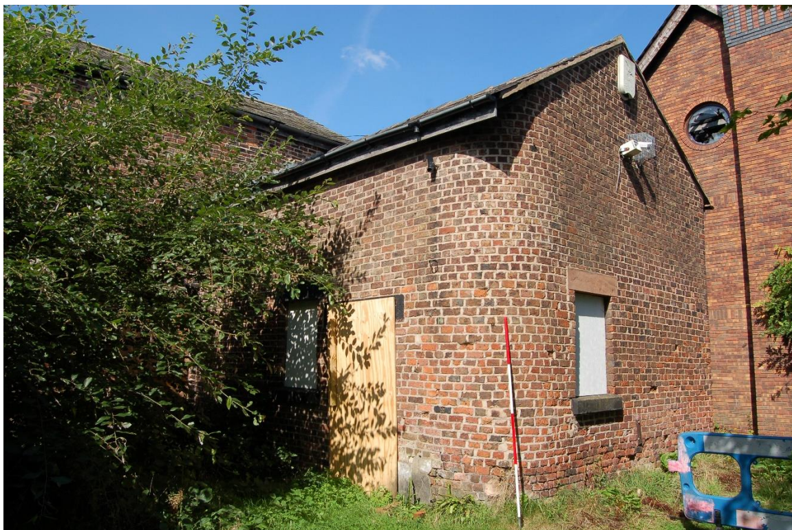
2. Main barn, west facing elevation of south-eastern adjoining single storey barn (F8D)
