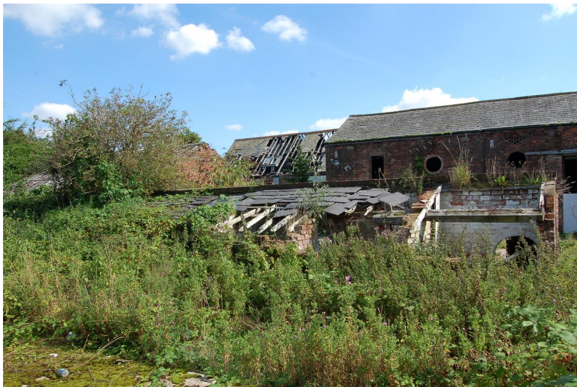
13. North facing elevation of pigsty
