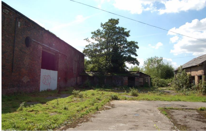
xi. General shot of farmyard with main barn (F8), attached northern lean to, and storage barn (F6)
