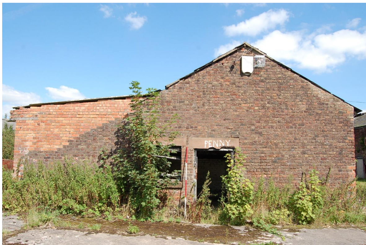
18. West facing elevation of storage barn
