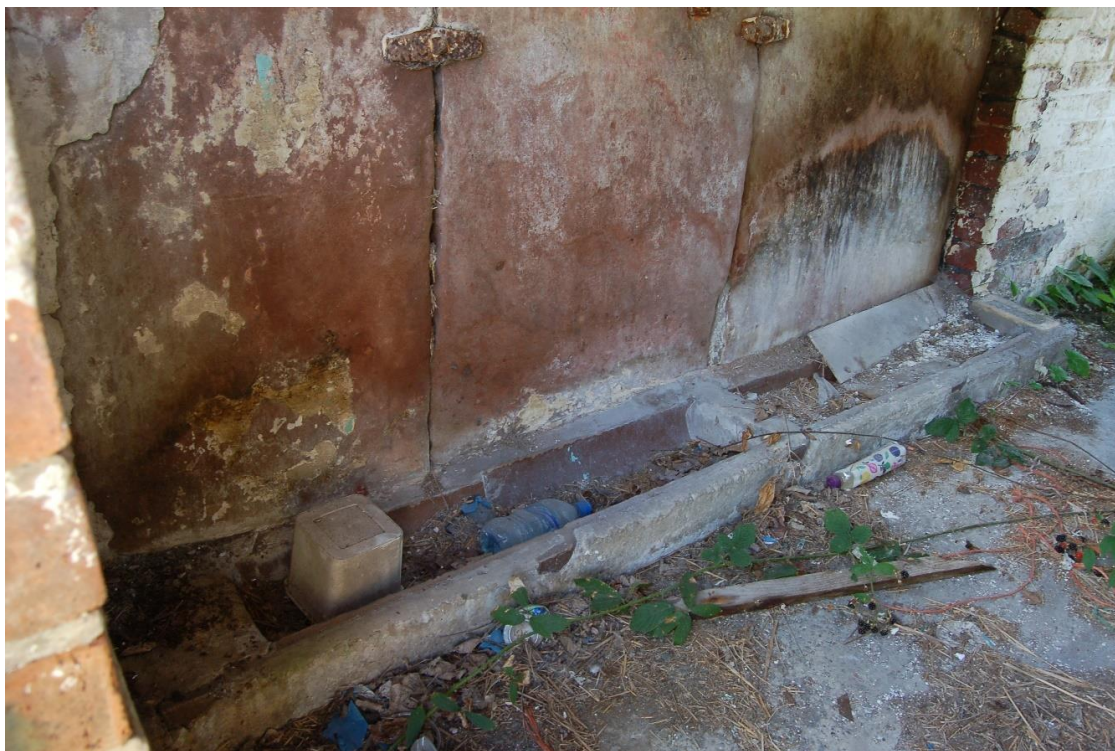
ii. Pigsty (F7) trough and wall between stalls
