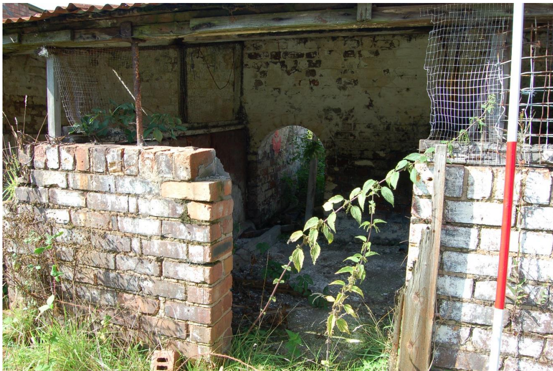
i. Interior, pigsty (F7) (south facing elevation)
