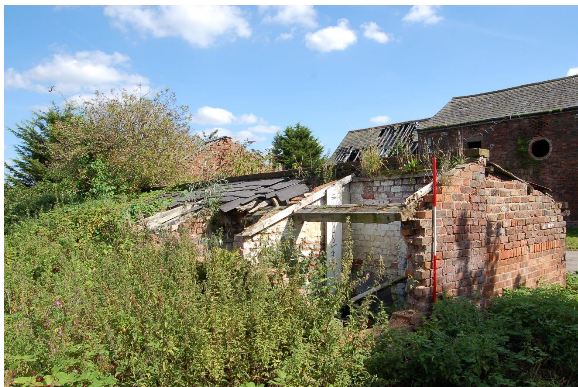
14. West facing elevation of pigsty
