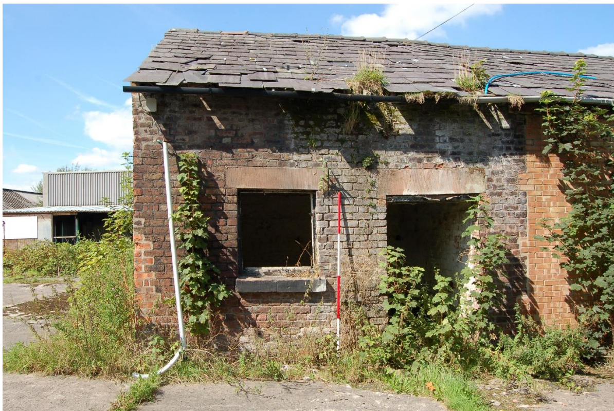
19. South facing elevation of storage barn
