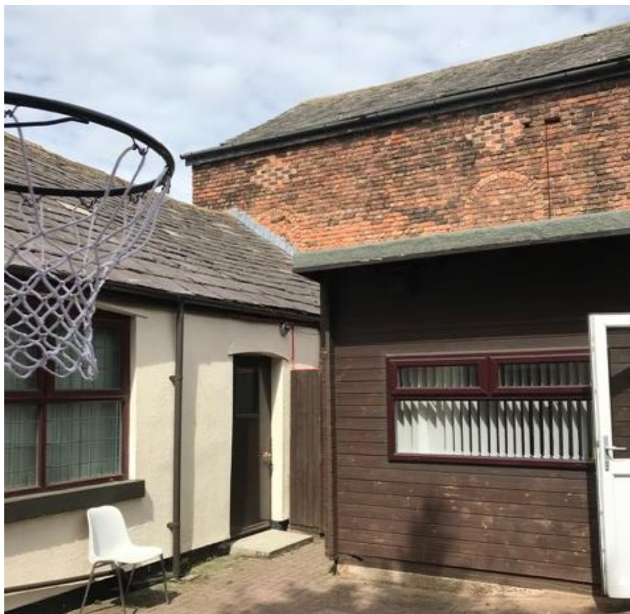
ix. Main barn south facing elevation from within the school grounds, with the attached southern eastern barn and modern wooden lean-to (Building B1)
