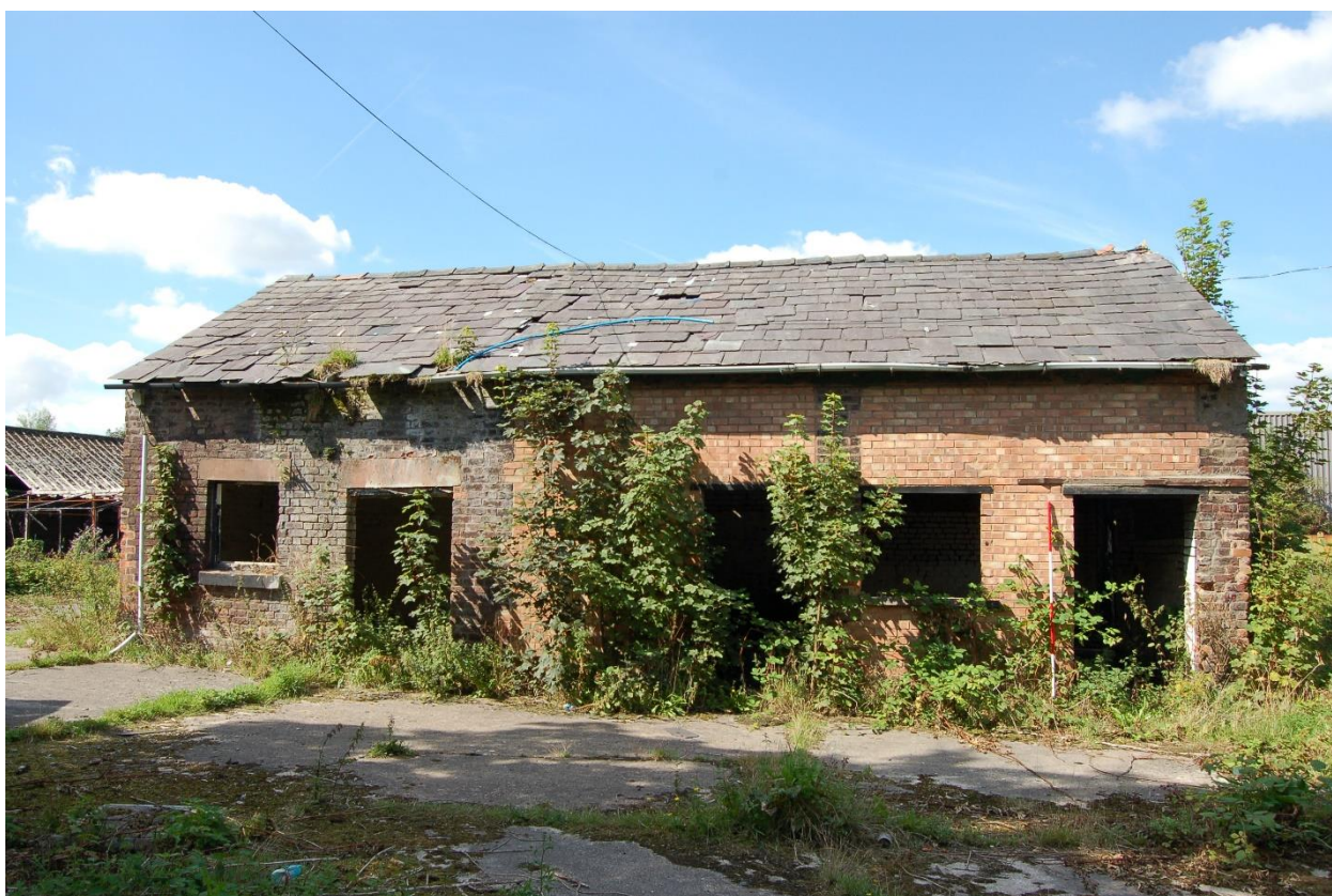
20. South facing elevation of storage barn
