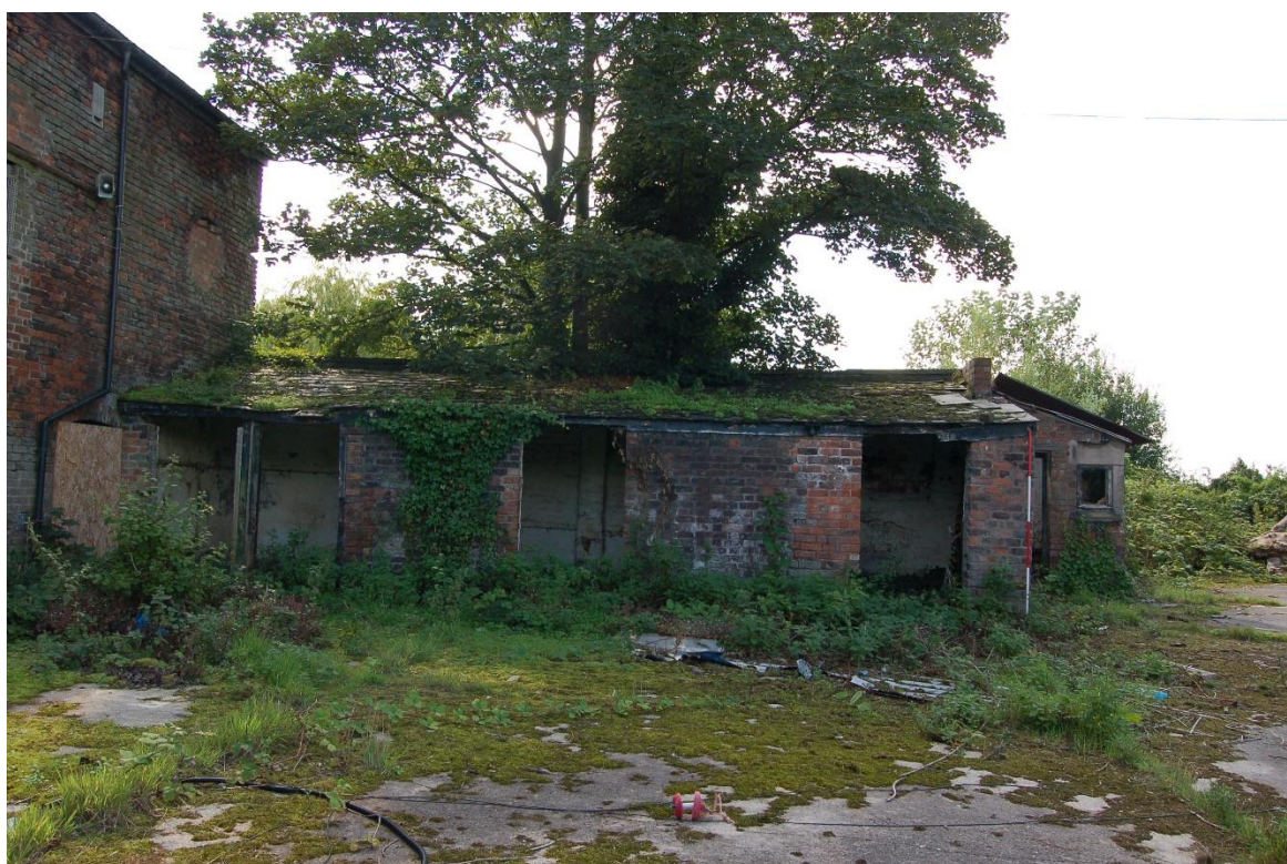
8. Attached single story lean-to (north side of main barn) (F8C)
