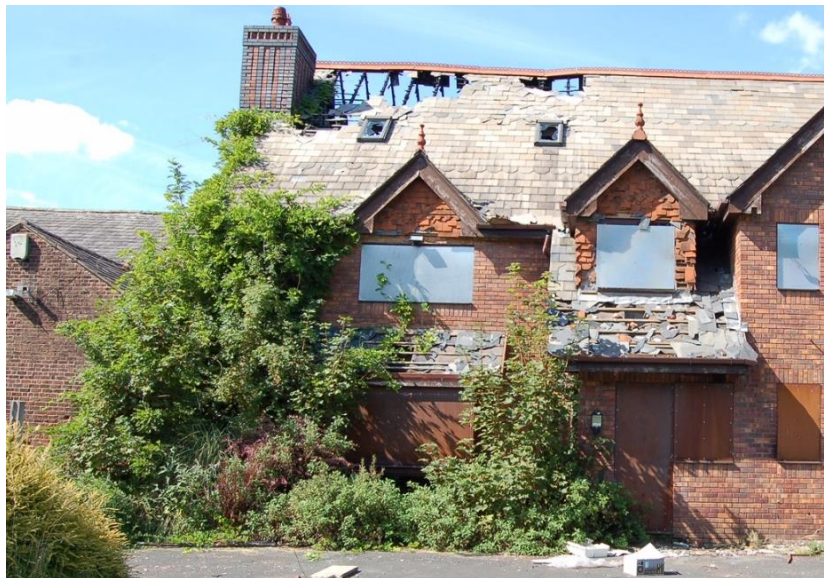
xii. Modern farmhouse with main barn (F8), south facing gable end of southeastern attached barn showing
