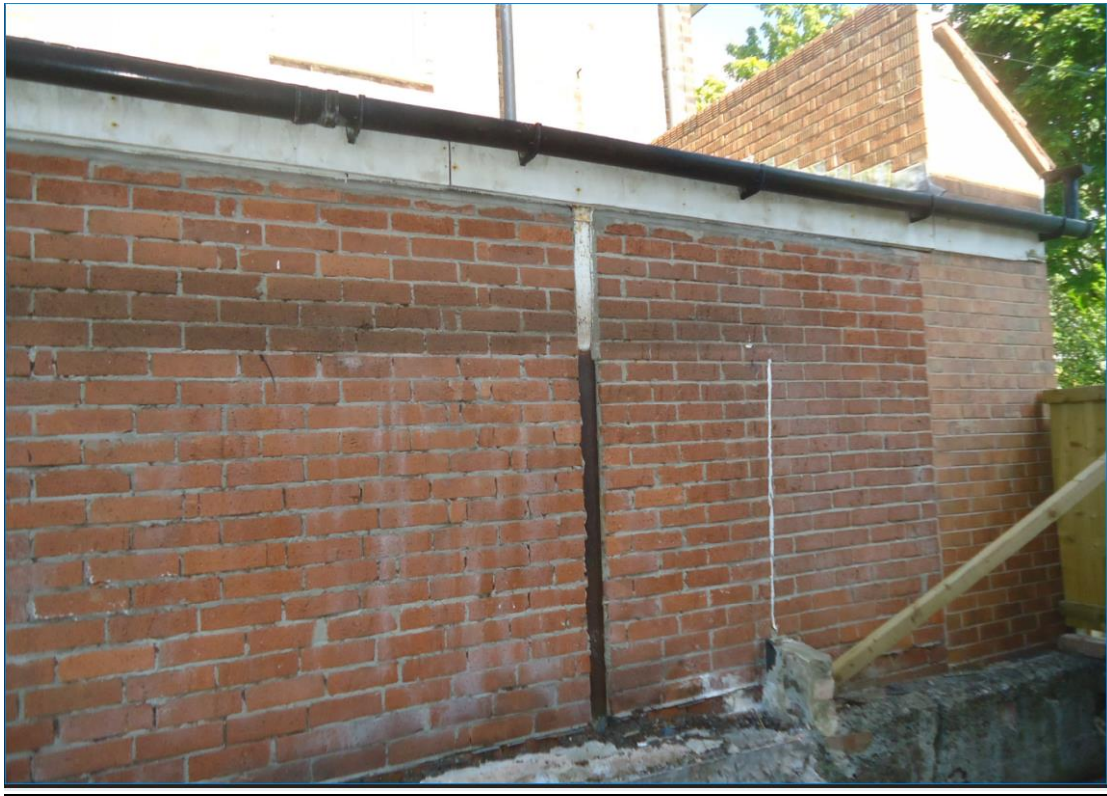
Boundary with No. 62 Bowring Park Avenue
