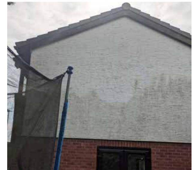
Existing gable end ( extension 2007)
