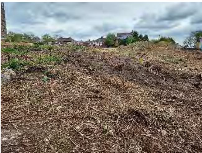
Figure 9 – Stockpiled soils in the central site section, looking north-west.
