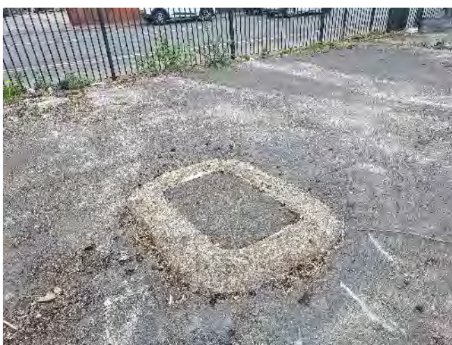
Figure 5 – A suspected disused service or on-site street light structure, looking north-east.
