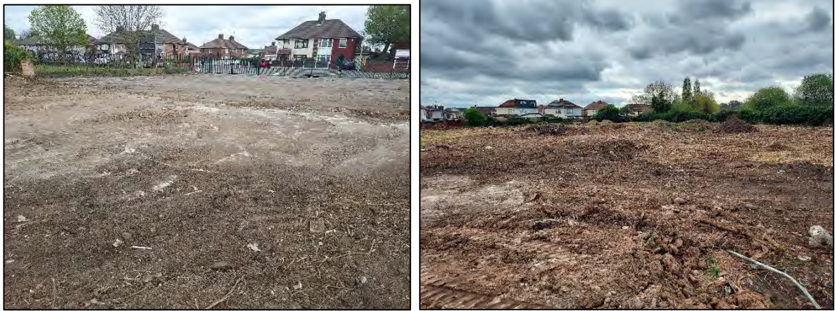
Figures 3 and 4: The northern site section (left) and the south-western site section with stockpiled soils (right).
