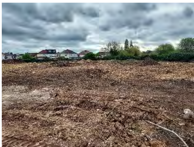
Figure 15 – The southern site section, looking south-east.
