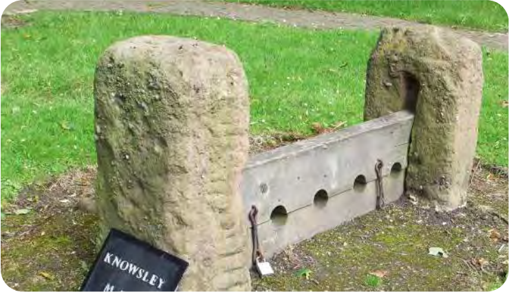
Cronton Stocks - Grade II Listed Building
