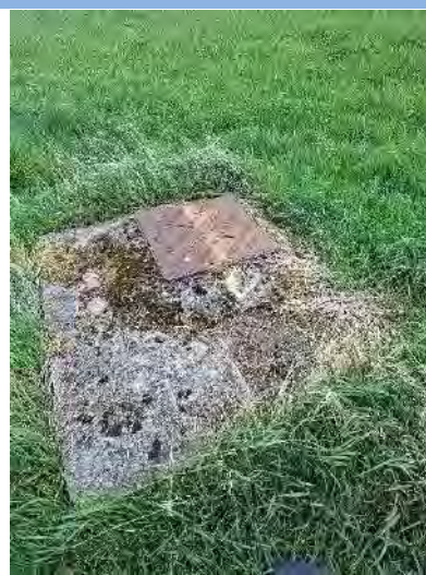
Photograph 6: Manhole in northern field in centre.
