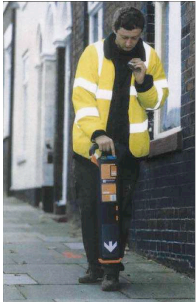
Figure 5 Using a cable locator
