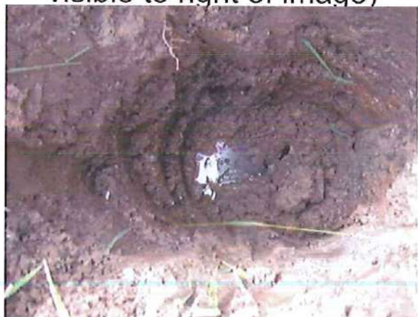
HDP02 excavation (black duct visible)
