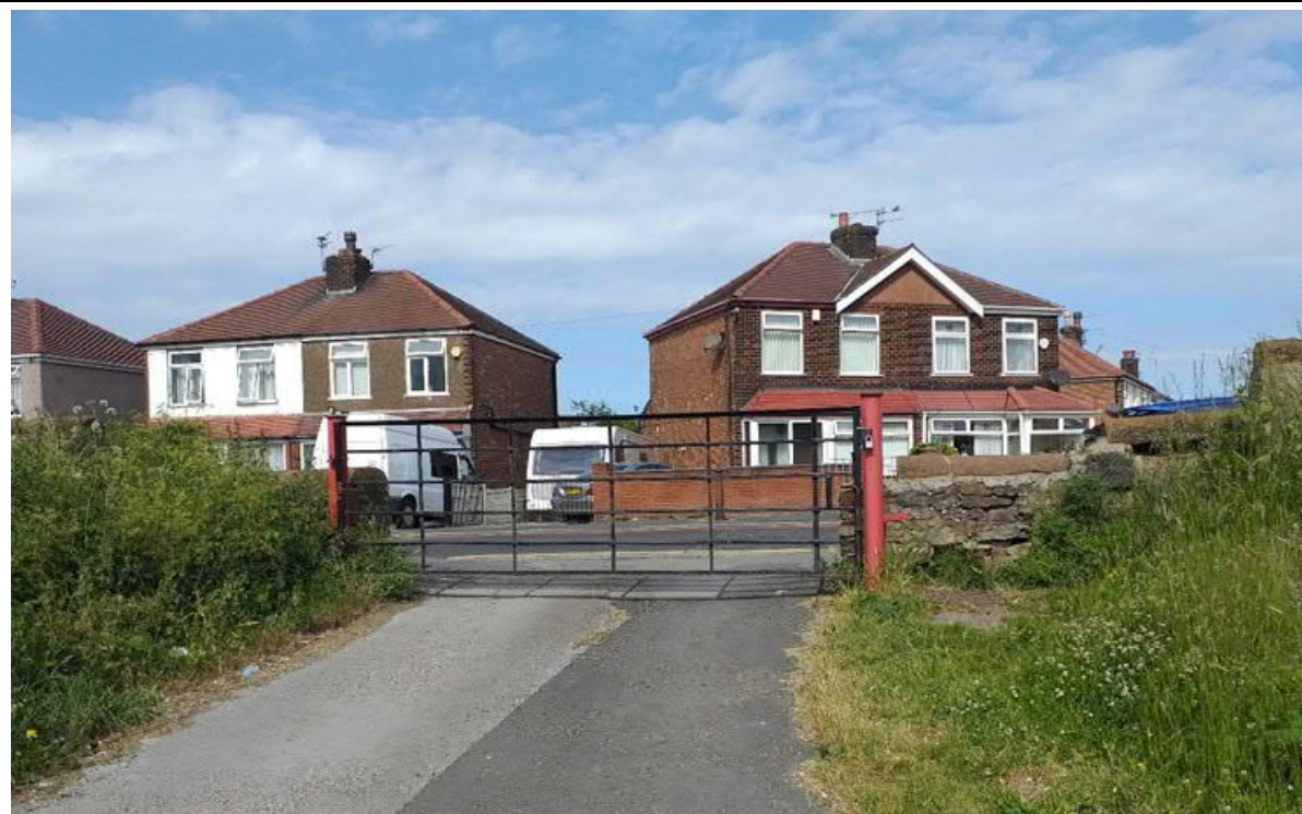
Photo 4: Gated vehicle access from Windy Arbor Road. Evidence of scarring presented by asphalt surface indicating past repair (photograph taken facing west).
