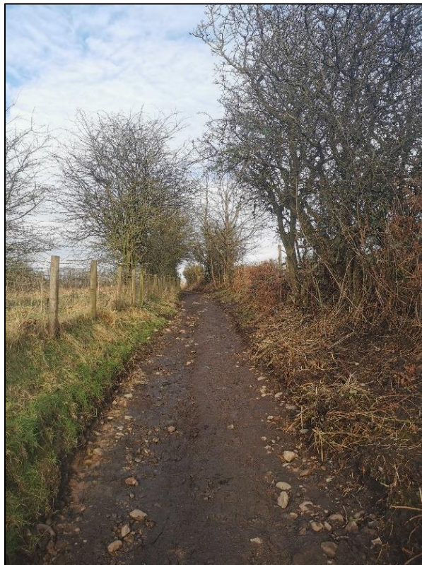
Photo 8: View north east showing Dobb Brow Road contained within the site area.
