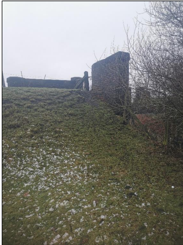
Photo 15: View west showing the historic railway bridge embankment.
