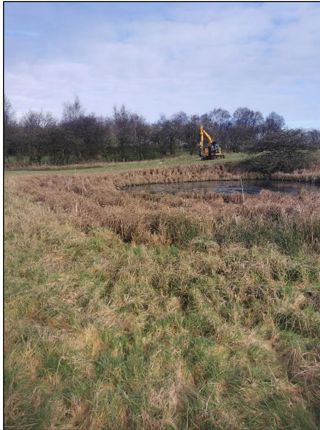
Photo 5: View north west showing the pond in the northern site section and the northern site boundary.
