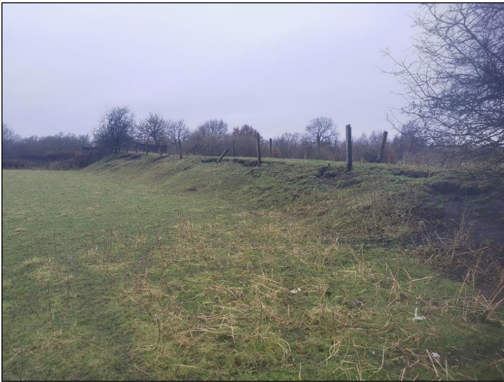
Photo 18: View north showing the historic railway bridge embankment.
