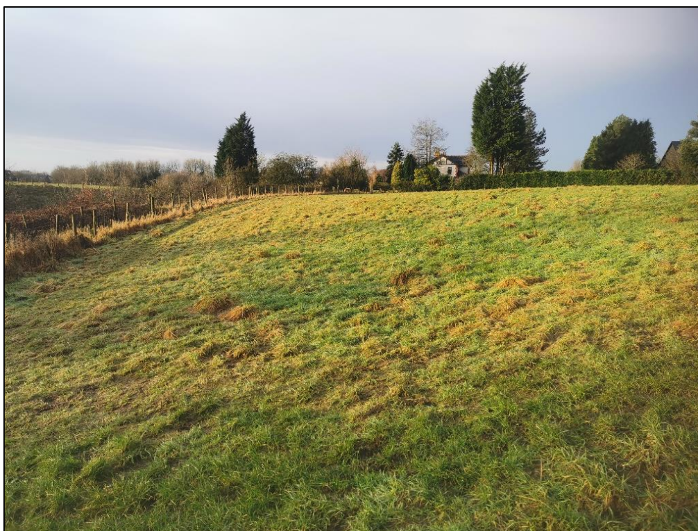
Photo 21: View south west in the south eastern site corner showing a natural slope.
