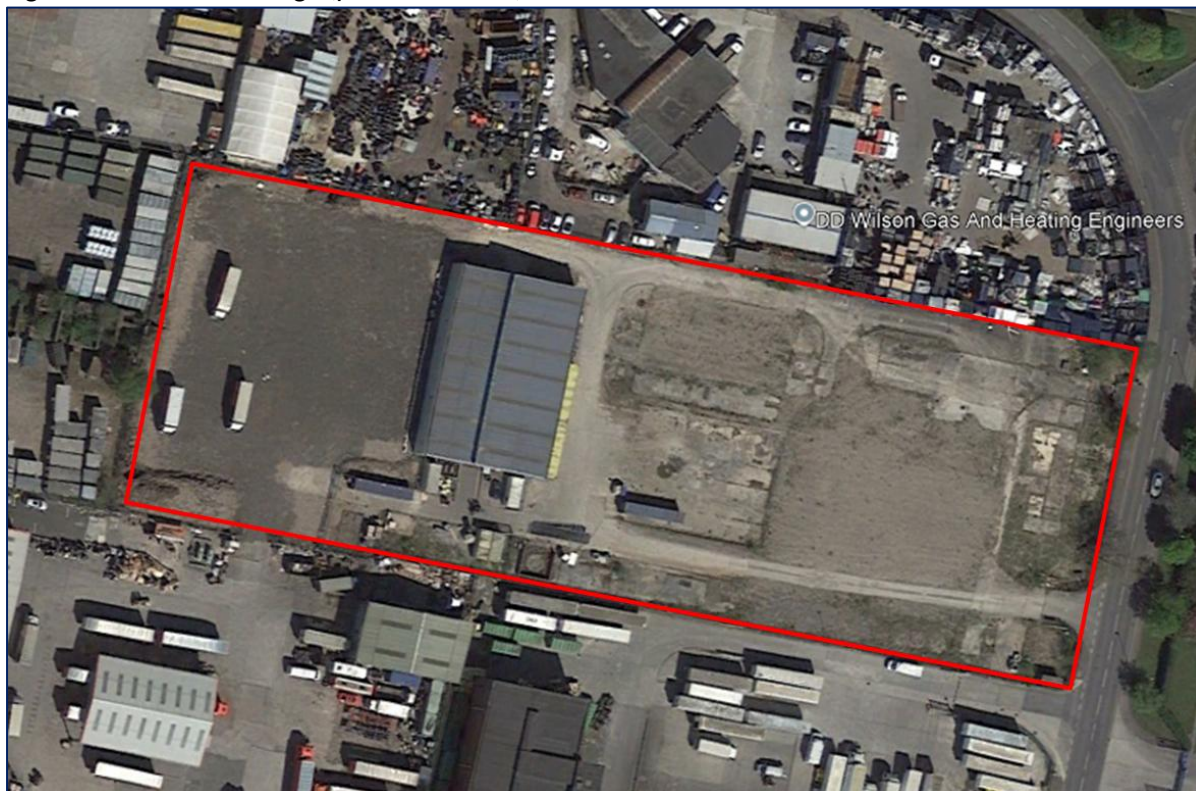
Figure 2: Site Aerial Image (pre-demolition)
