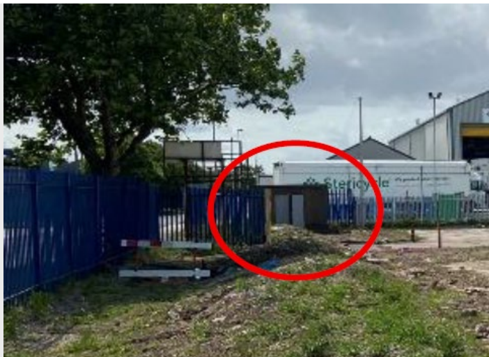
Photograph 5: Structure of building B2 with negligible roosting potential in relation to u1b6 and u1c habitats on site.
