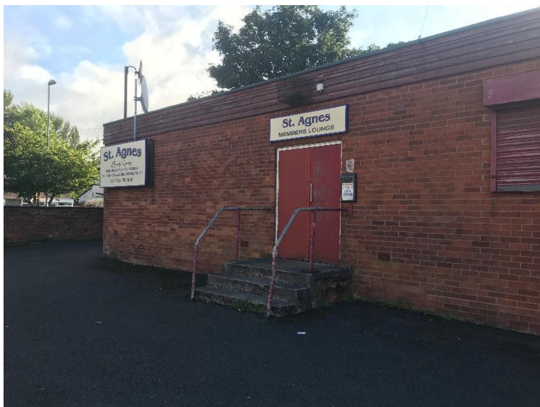
Plate 2 – West facing elevation of the club
