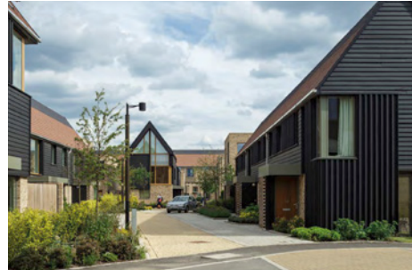
① Timber to First Floor Accommodation
