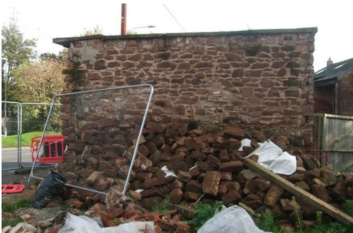
Figure 3: Still-standing portion of original wall, perpendicular to section requiring reconstruction (at left)
