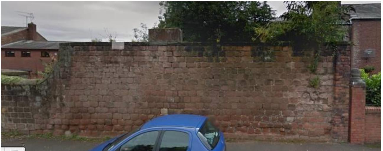
Figure 4: Original appearance of front elevation of currently dismantled boundary wall (image: Google Streetview)
