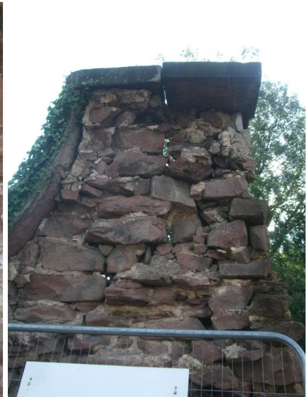
Figure 2a-d: Evidence of deterioration in still-standing sandstone boundary wall
