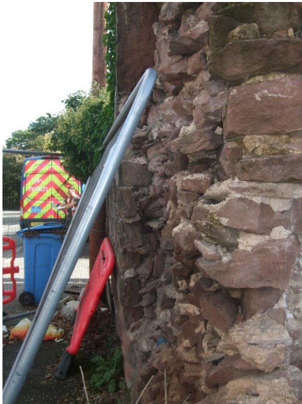
Figure 2a-d: Evidence of deterioration in still-standing sandstone boundary wall
