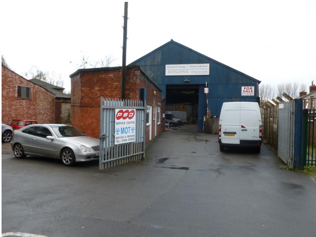
VIEW OF SITE ACCESS
