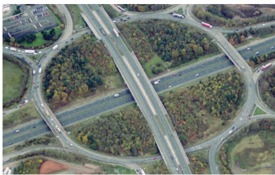
10. Ring Road serving M62 Motorway
