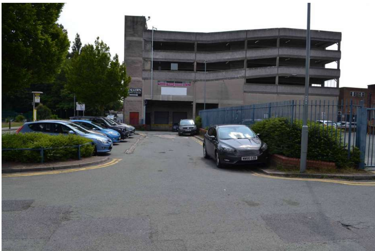
Plate 79: Sightline to the south across the ground level car park adjacent to Lathom Road, towards the north-facing elevation of the Lathom Road Car Park.
