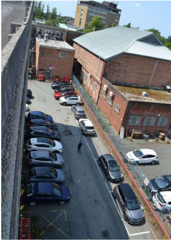
Plate 73: Sightline to the west from the roof the Lathom Road Car Park to the ground level car park/service yard to the rear (east) of the retail units on Cavendish Walk.
