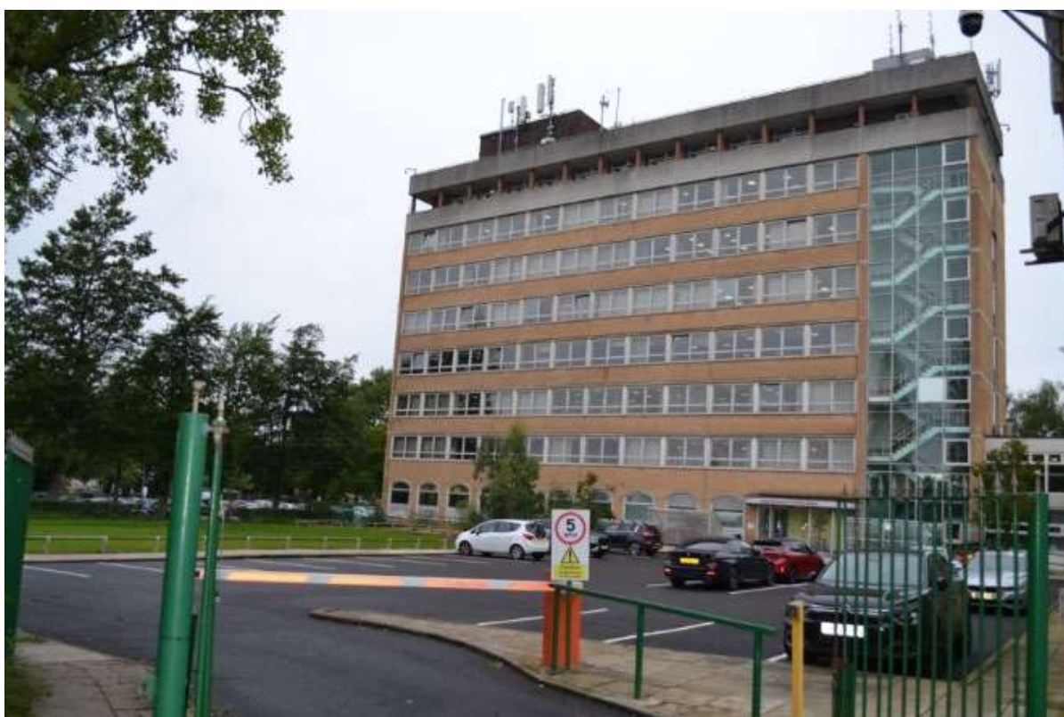
Plate 56: Sightline to the north-east highlighting the south-west facing elevation of the Council Municipal Building.
