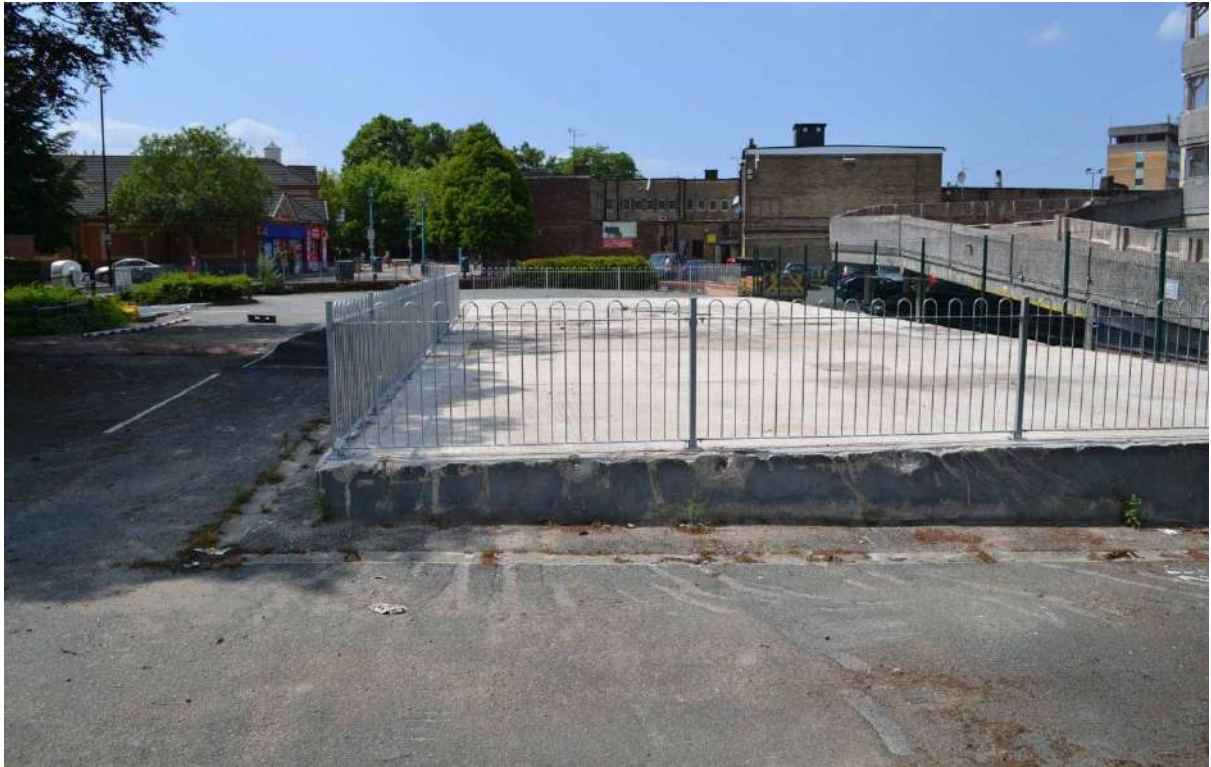
Plate 75: Sightline to the west over the now cleared site of the four-storey Ingeus office. This was the site of a Victorian villa.
