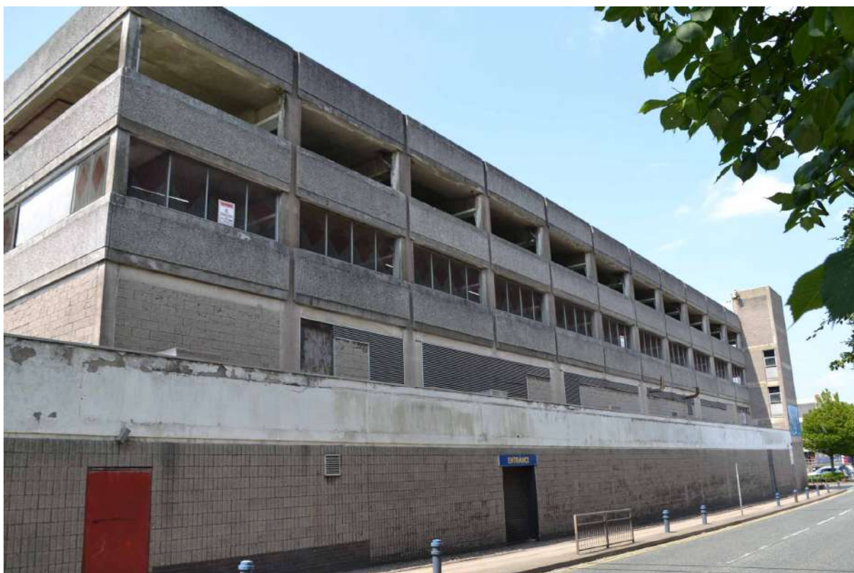
Plate 34: Sightline to the north-west from Lathom Road showing the east-facing elevation of the Lathom Road car park.
