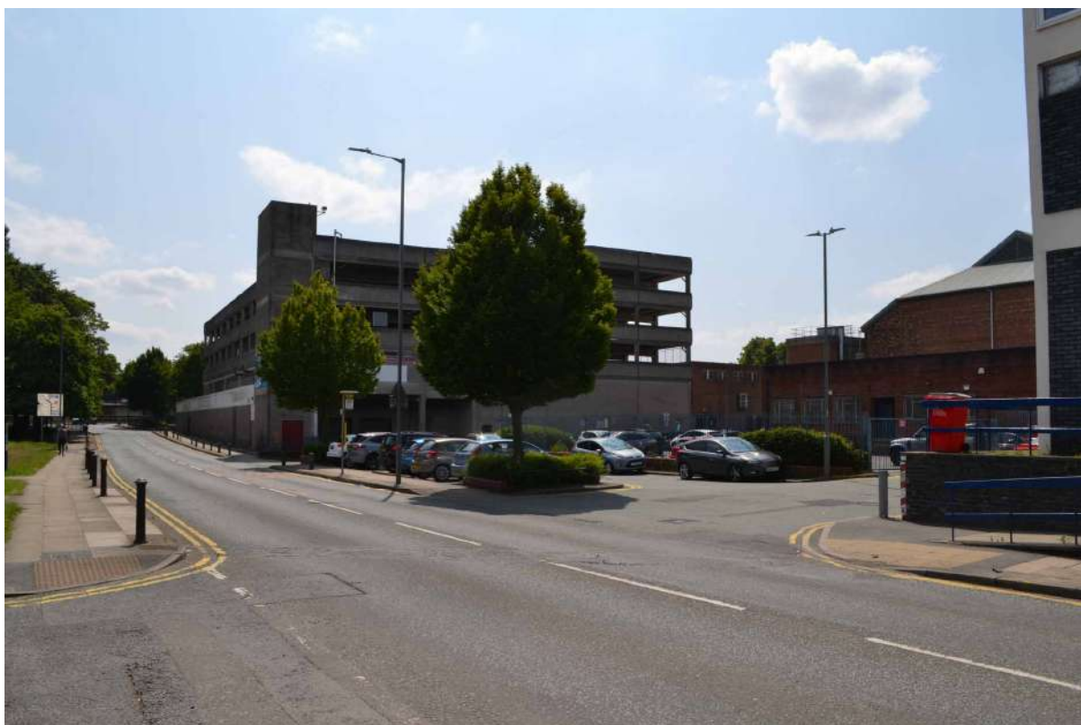
Plate 31: Sightline to the south-west along Lathom Road towards the Lathom Road car park Site.
