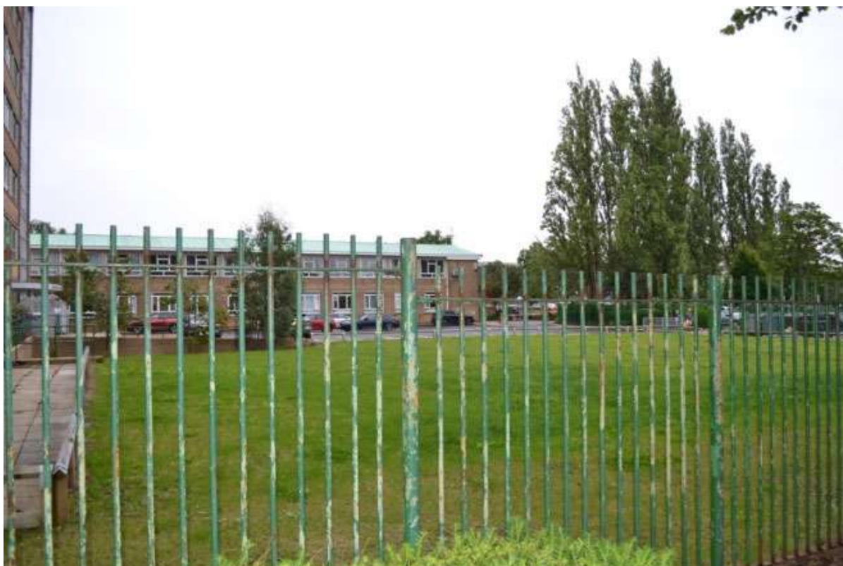
Plate 47: Sightline to the south-east across the lawn to the south-west of the Council Municipal Building.
