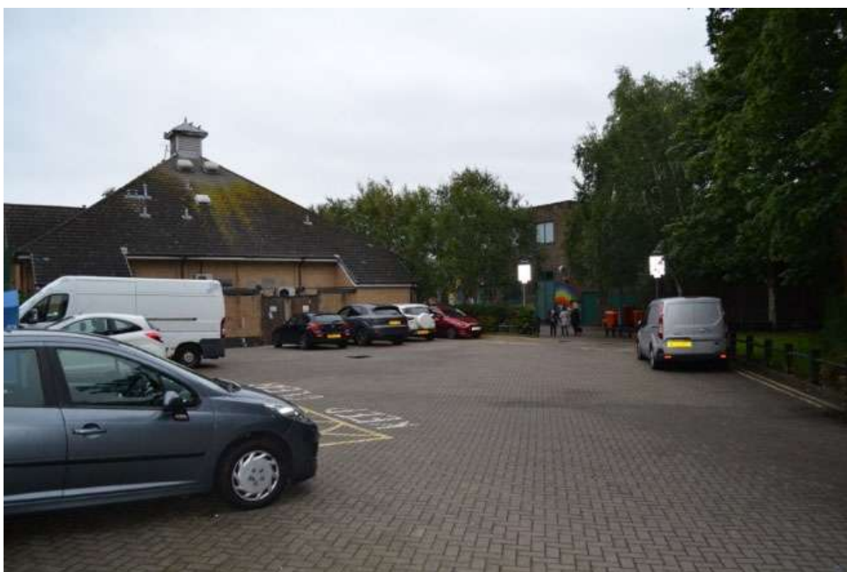
Plate 50: Sightline to the south-east towards the rear elevations of retail premises on Derby Road.
