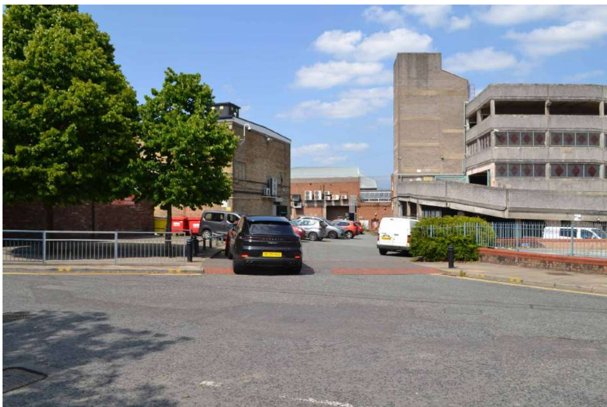
Plate 80: Sightline to the north from Huyton Hey Road towards the service yard to the rear (east) of the retail units on Cavendish Walk. This was the site of a Victorian villa.
