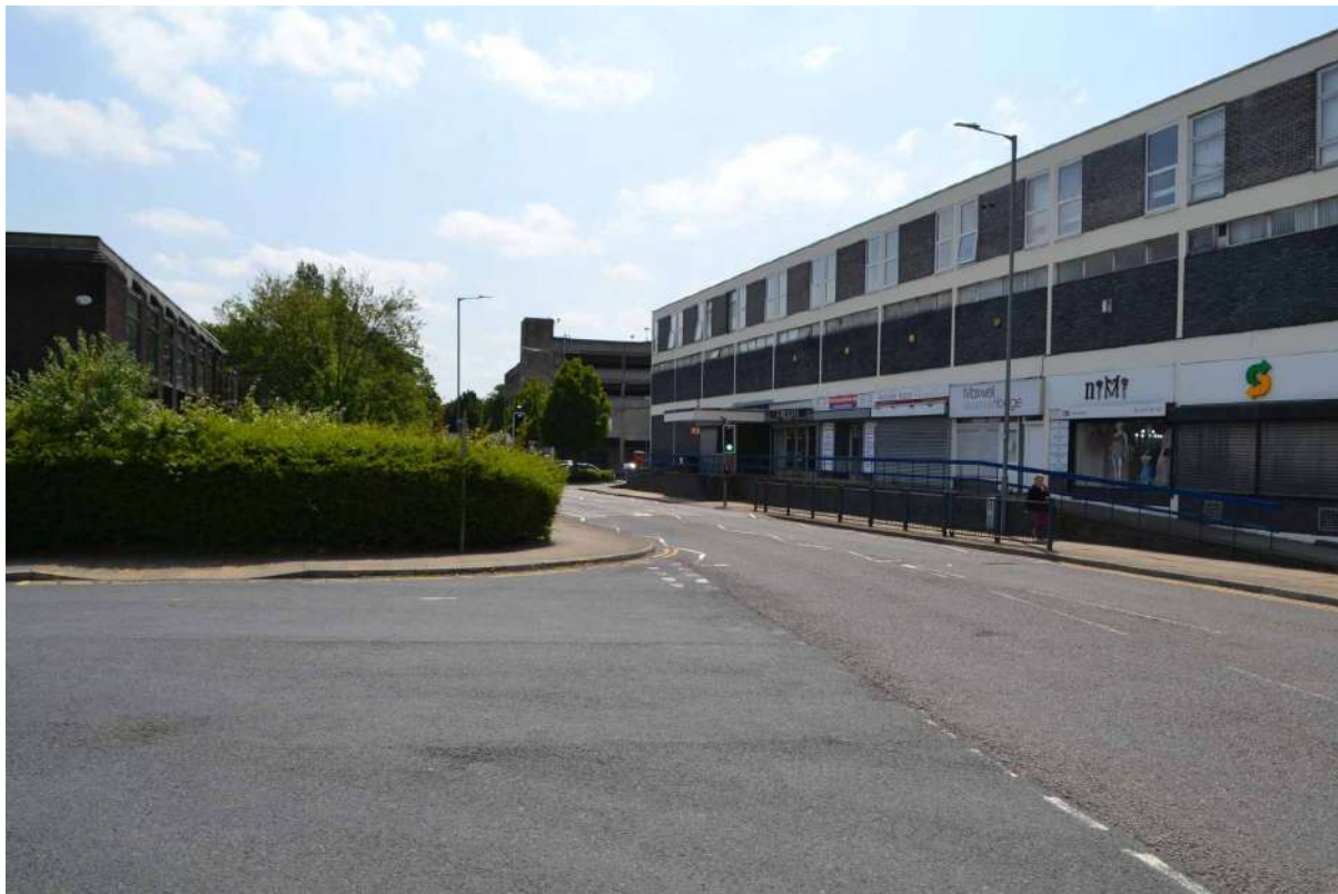
Plate 30: Sightline to the south-south-west along Lathom Road towards the Lathom Road car park Site.
