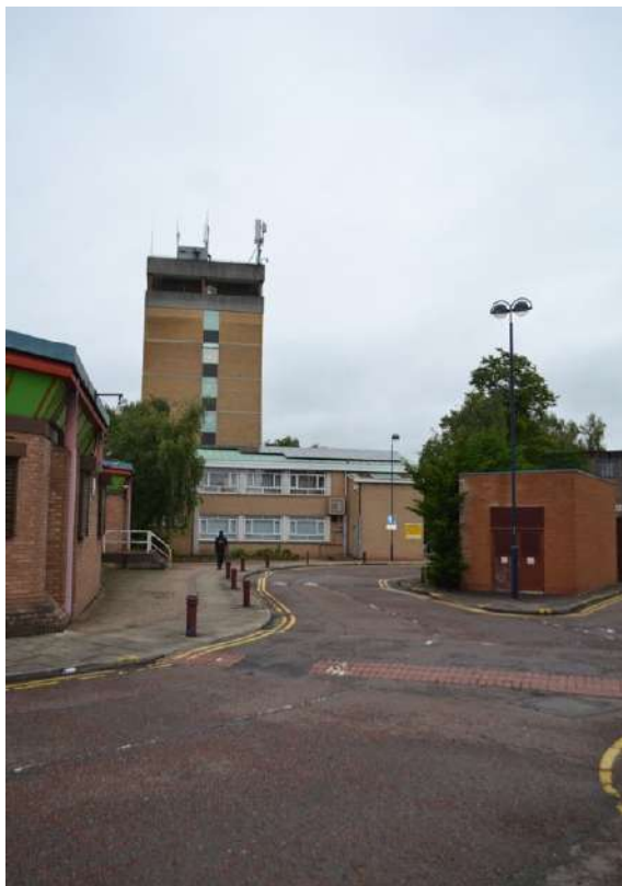
Plate 20: Sightline to the north along Westmorland Road with the north-facing elevation of the Council Municipal Building prominent.
