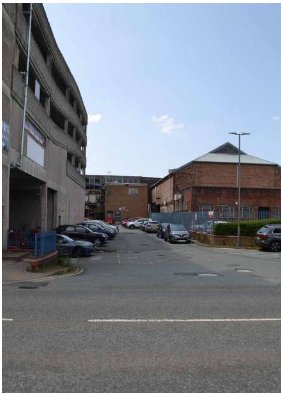
Plate 76: Sightline to the west from Lathom Road to the ground level car park/service yard to the rear (east) of the retail units on Cavendish Walk. The north-facing elevation of the Lathom Street Car Park is to the left.
