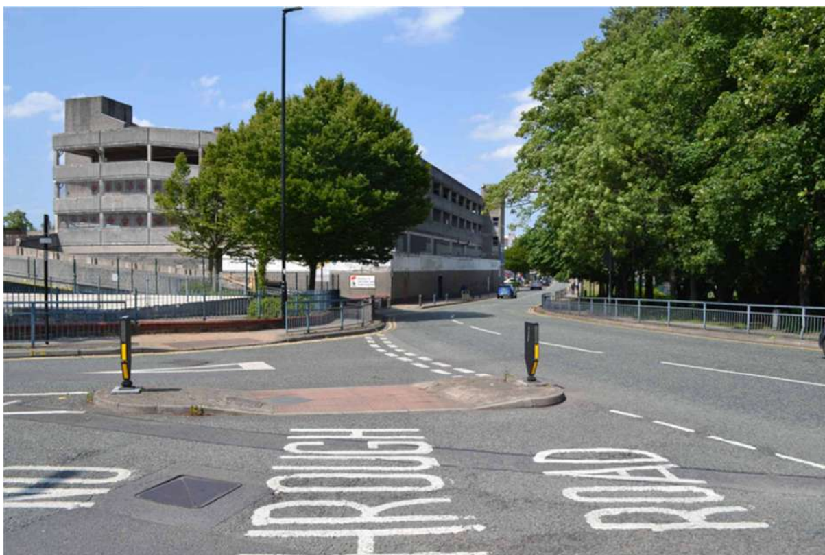
Plate 36: Sightline to the north-west from the junction of Huyton Hey Road and Lathom Road towards the Lathom Road car park Site.
