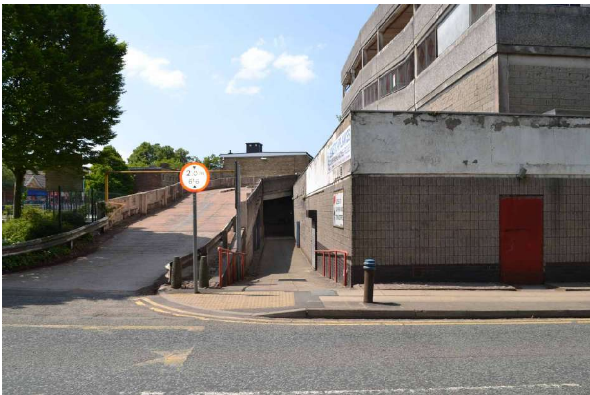
Plate 33: Sightline to the west across Lathom Road towards the ramp into the Lathom Road car park and the pedestrian underpass providing access to Cavendish Walk.
