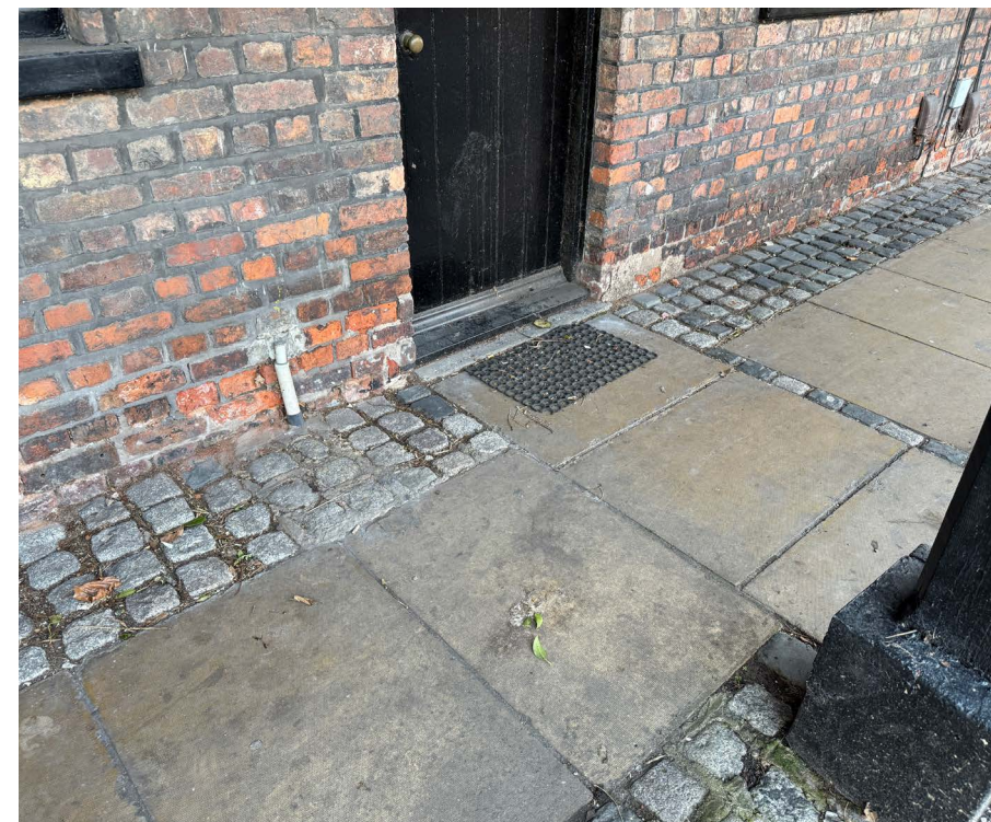
Figure 2.35: Surface treatment to Bluebell Lane
