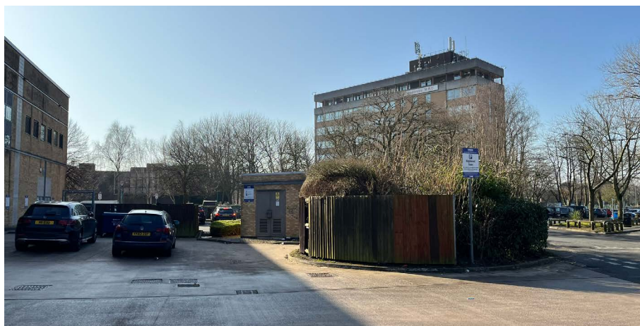
Figure 1.11: 8 | Service yard and sub station to rear of Cavendish Walk
