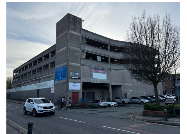
Figure 1.14: 11 | Multi-storey car park on Lathom Road
