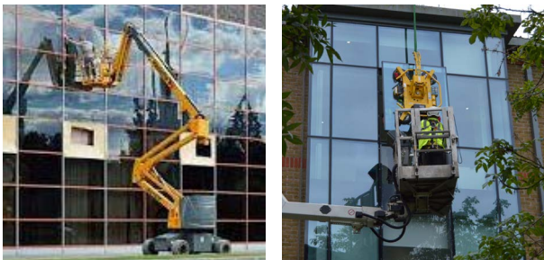
Facade access/ window replacement using MEWP systems
