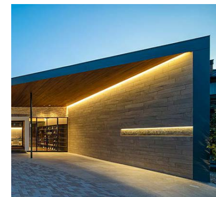
LED Strip lighting to feature entrance
