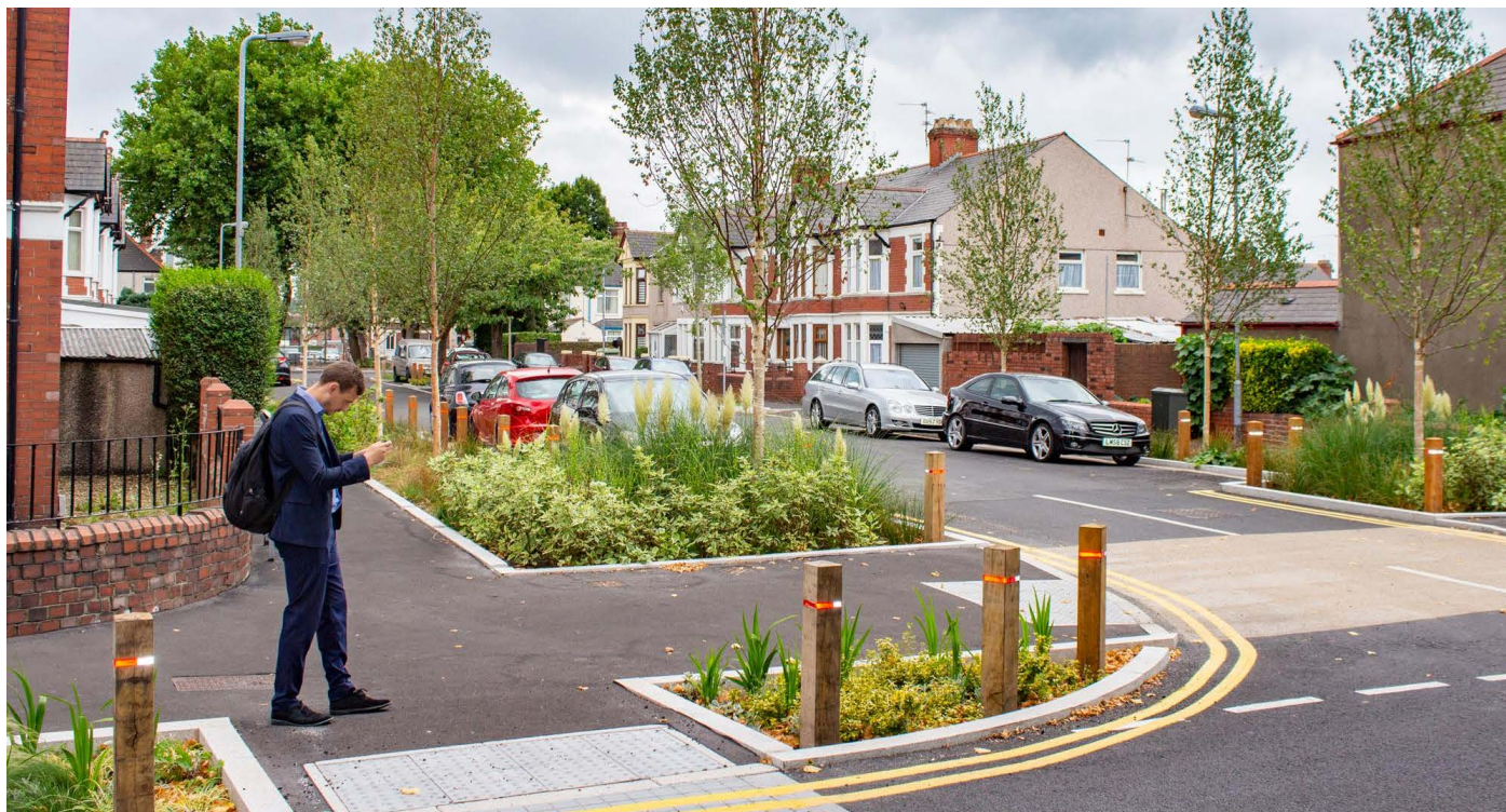
Figure 5.14: Greener Grangetown, Cardiff by GreenBlue Urban © GreenBlue Urban SuDS rain gardens integrated into the streetscape and public realm
