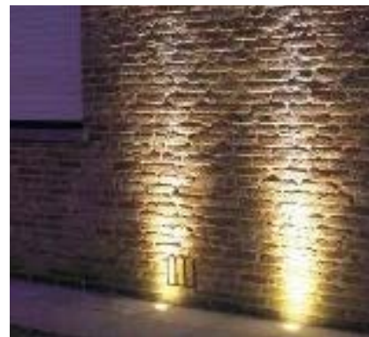
3. Example: Perimeter Building uplighters
