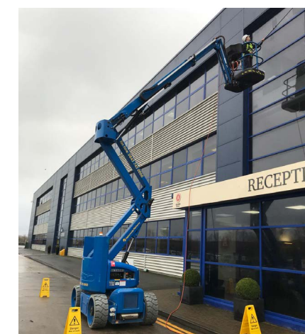
Facade Cleaning / maintenance via MEWP system
