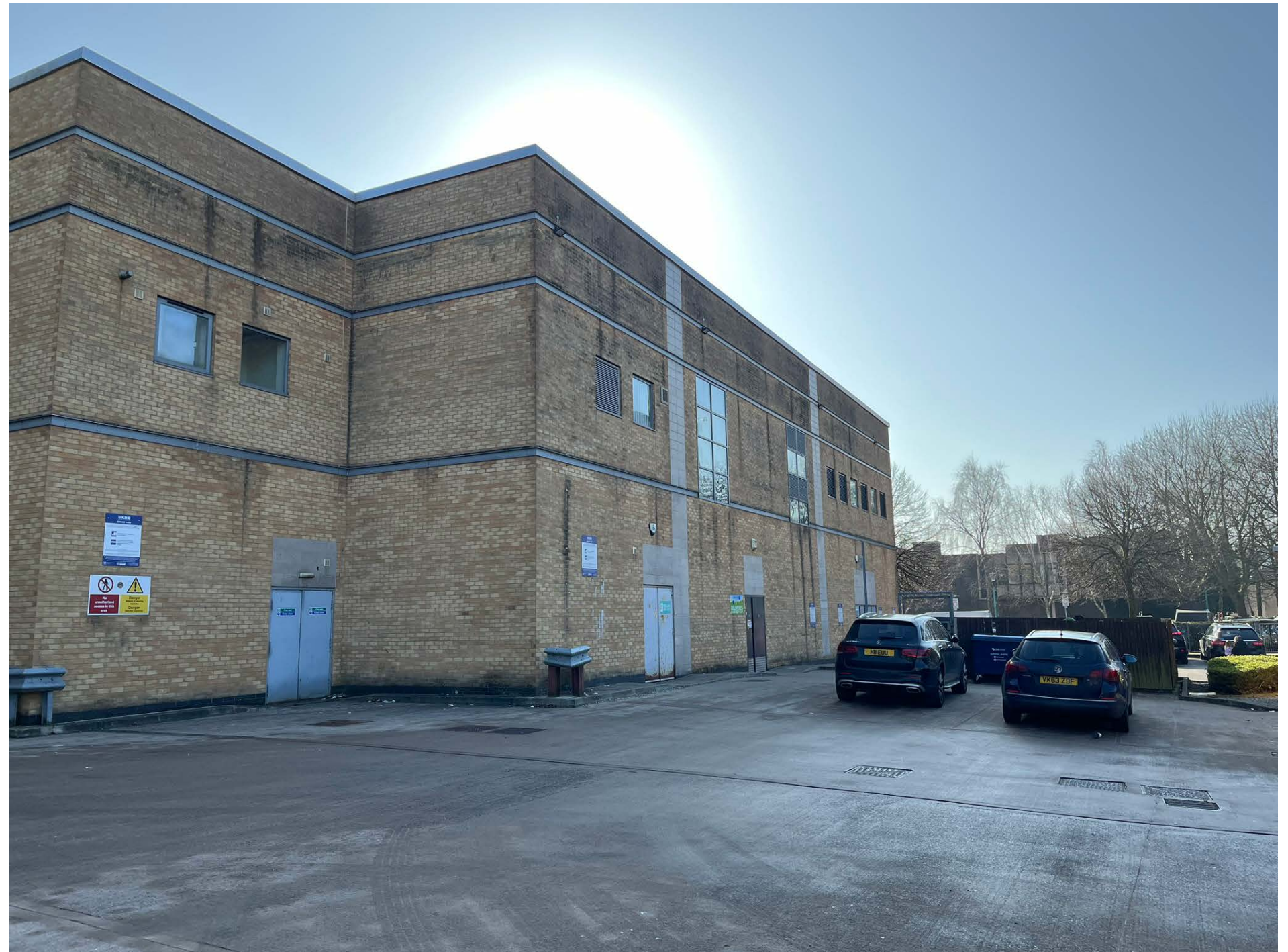
Figure 10.2: Cavendish House's service access fronts onto the site.
