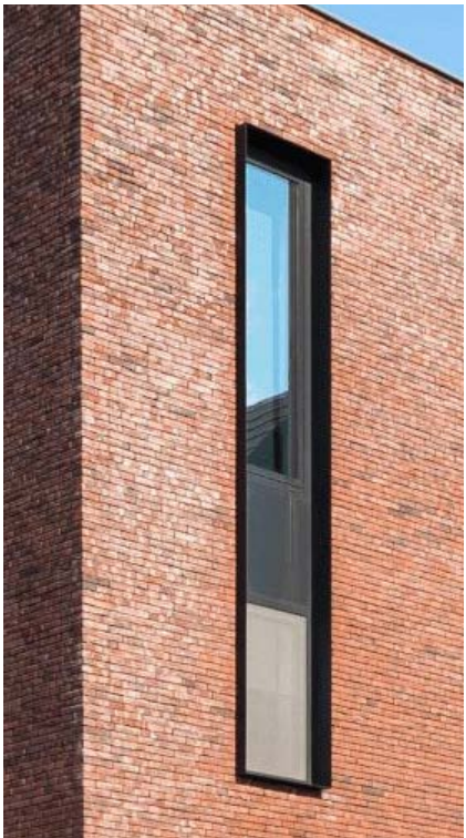
Detailing - Aluminium Window Surround
