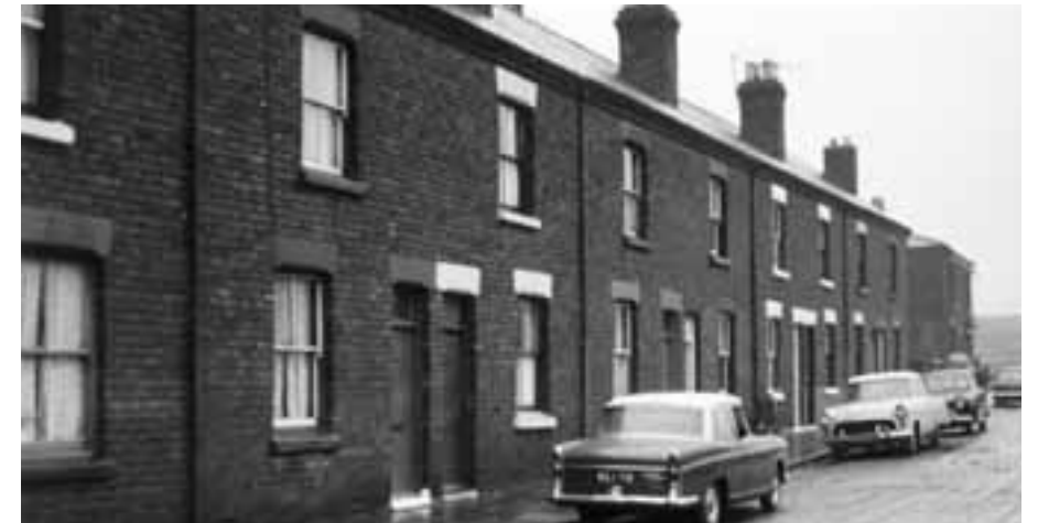
02. Terraced Factory Housing - Derby Street, Huyton Quarry
