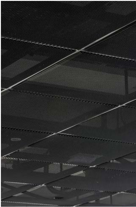
Metal mesh ceiling and exposed services
