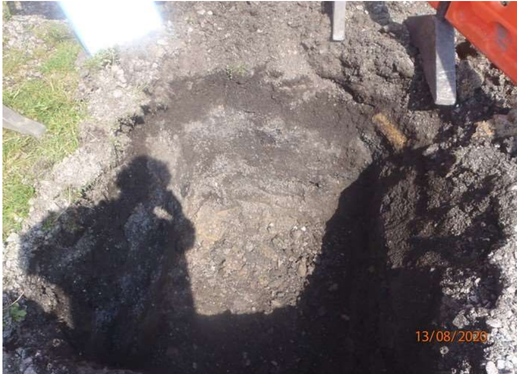
PHOTO 4 SHOWING SOAKAWAY LEVEL AT START OF 2nd DAY
