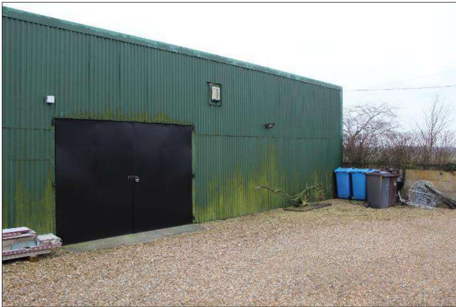
Plate 4: View of metal garage/store located on the site, looking west-southwest
