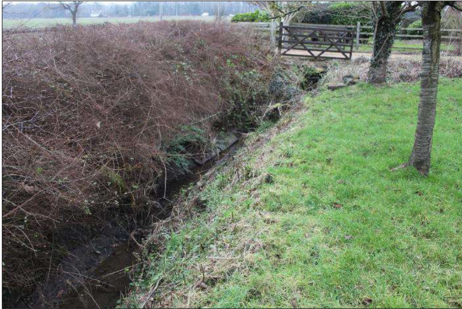
Plate 7: View of drain running under the site entrance, looking north
