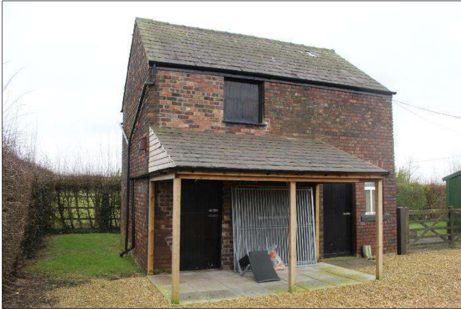
Plate 3: View of two storey red brick building on the site, looking south-southwest
