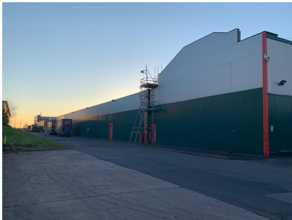
Northeast corner of the building showing profiled metal sheet cladding
