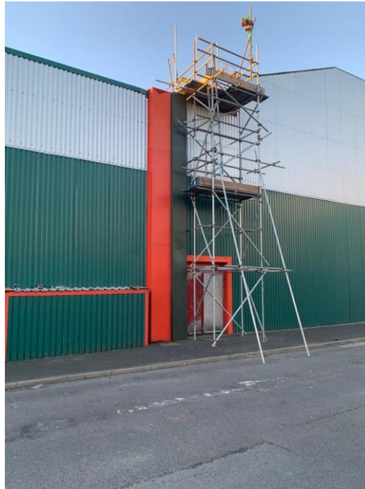
North elevation - Access for re-roofing works over substation area
