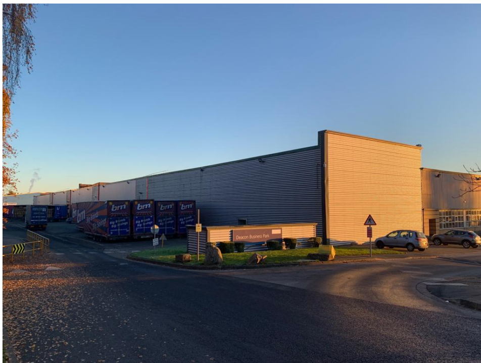
Northwest corner of the building where access for HGVs to the east elevation is apparent
