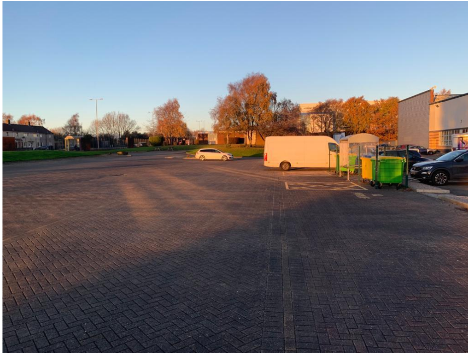
Extensive car parking facility to west elevation constructed of brick pavers (looking north)
