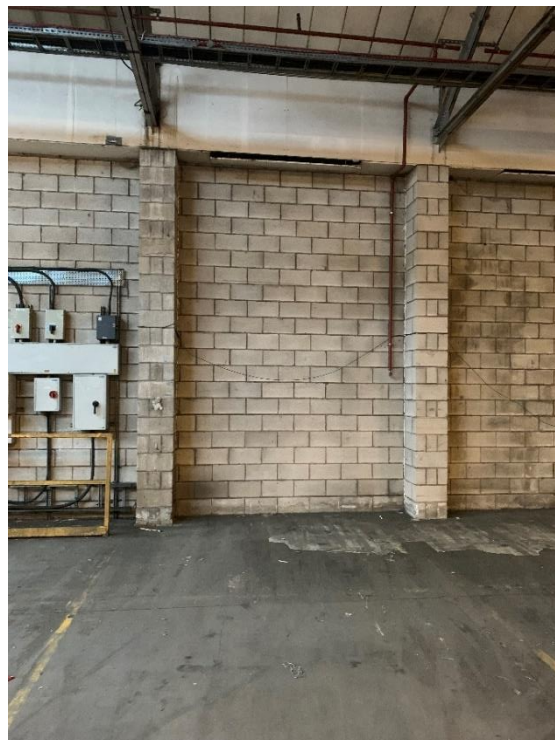
Internal west elevation fire wall
