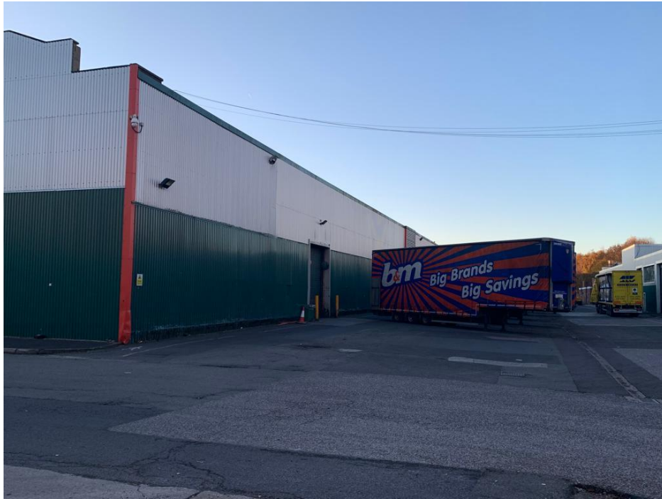
Tarmac hardstanding / access road to north elevation
