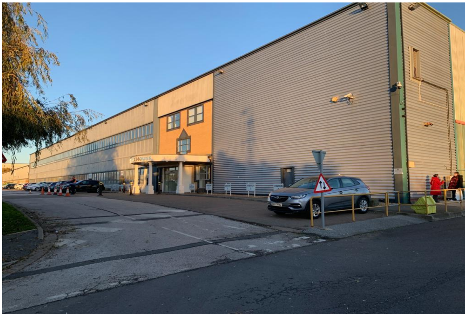
Southwest corner of the building showing car park egress arrangements and access to first floor offices through reception area
