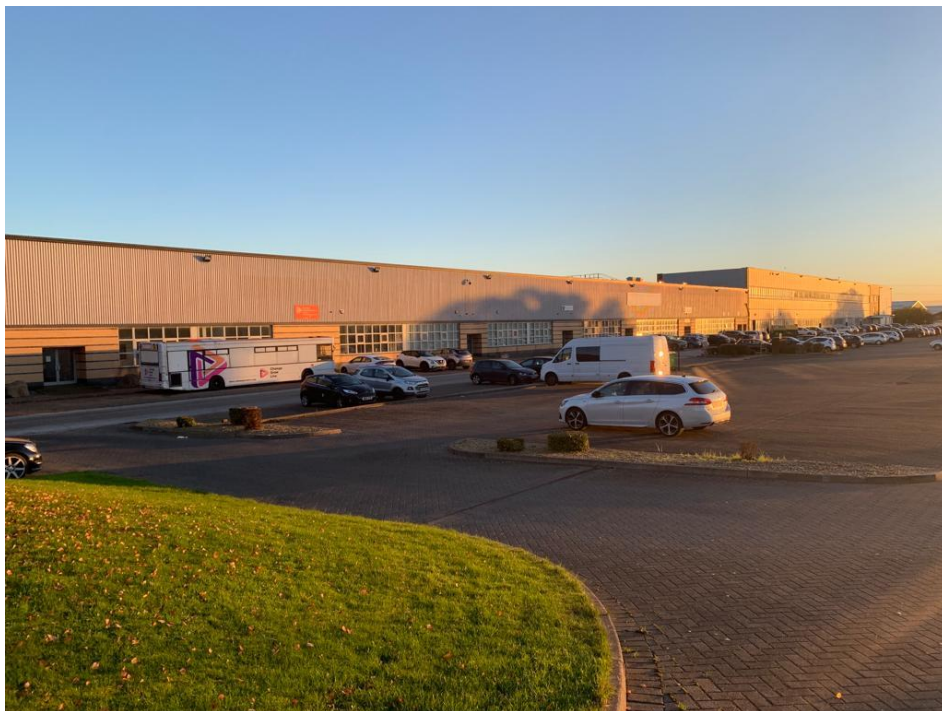
South elevation showing combination of upper profiled cladding over composite flat panel below
