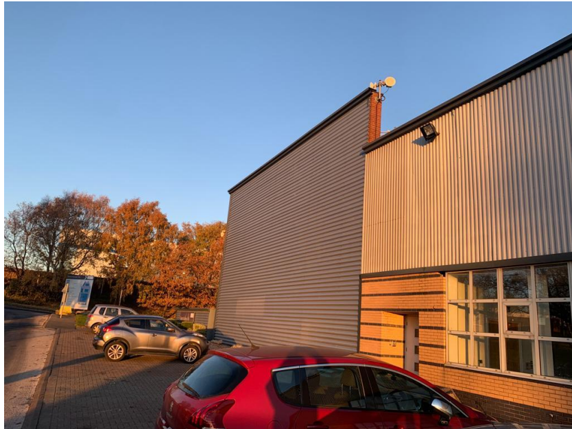
Northwest corner of the building where the building has been extended
