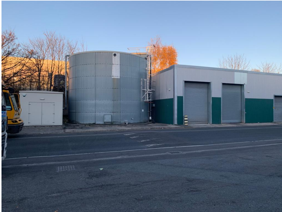
Sprinkler tank building to the northern boundary
