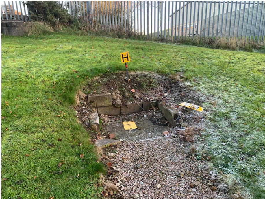
Fire Hydrant to East Elevation. Possible use for dust suppression during demolition
