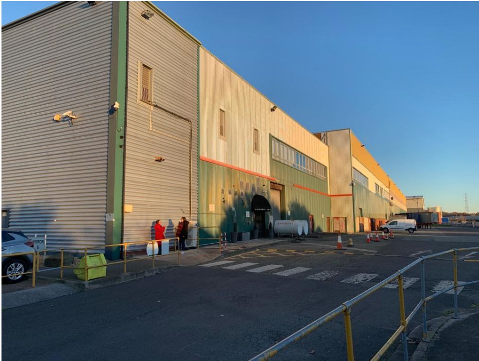
Southwest corner of the building depicting variance in cladding as building has been upgraded
