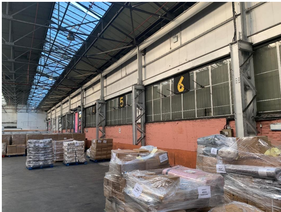
Laced columns to redundant crane rails
