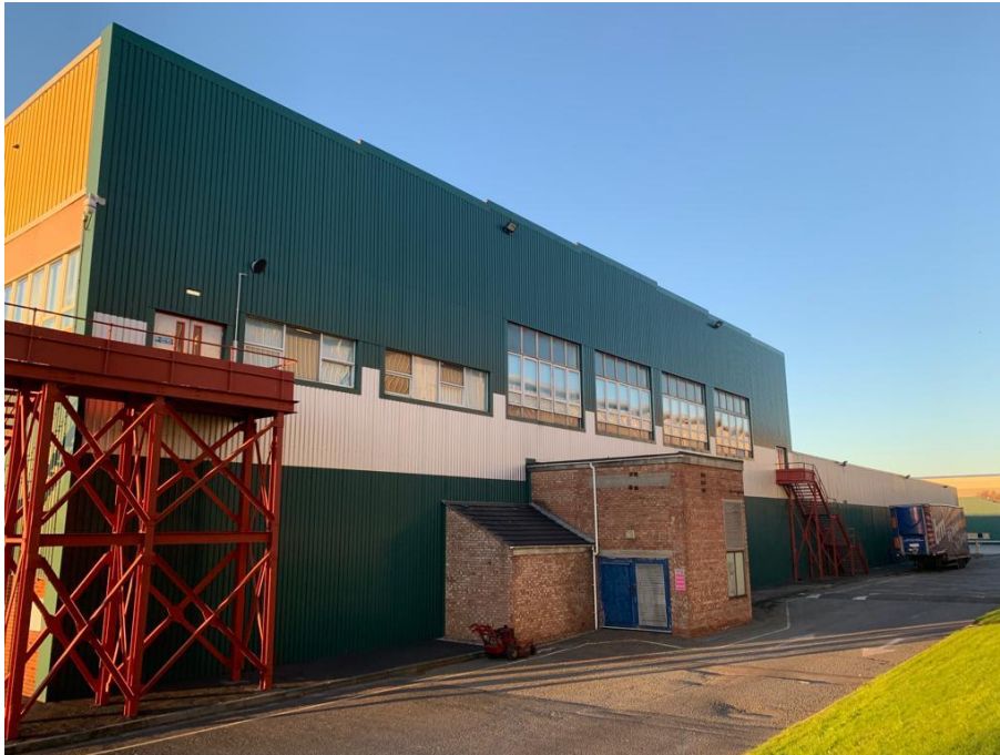
Southeast corner of the building showing fire escape stair to first floor offices
