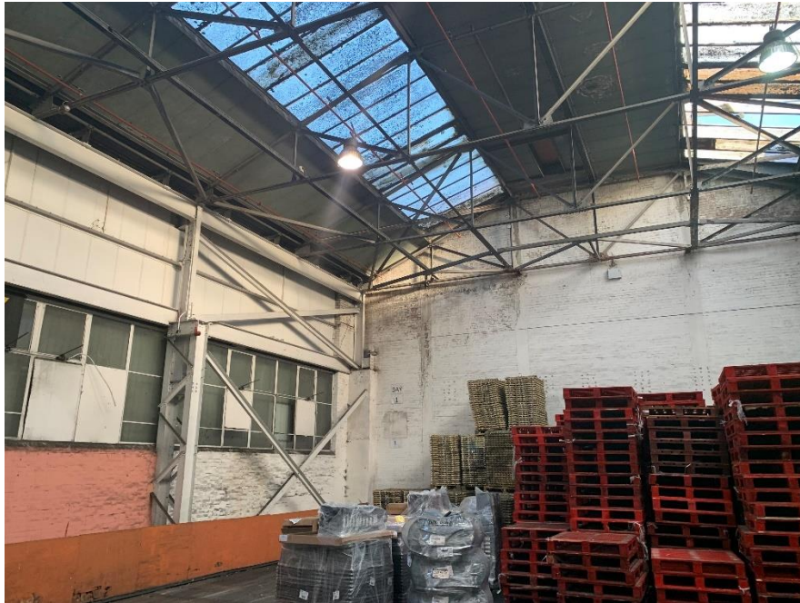
Northern end bay depicting laced columns to redundant crane frames
