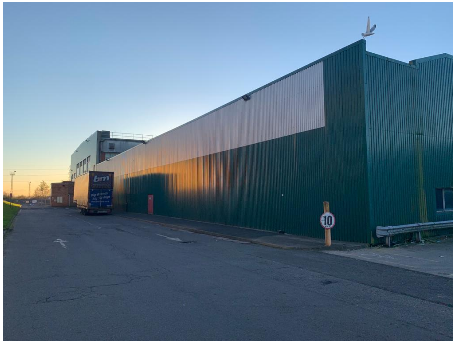
East elevation looking south west
