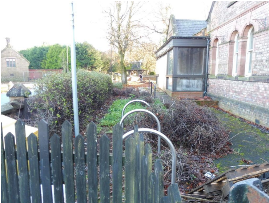
Photograph 9: View of hard standing to north facing (front) of building.
