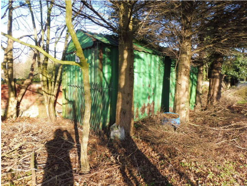
Photograph 7 View of metal shed outbuilding to south west corner of site.
