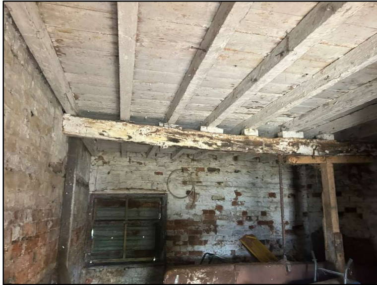
Photograph 3- taken from ground floor level showing 1 st floor structure
