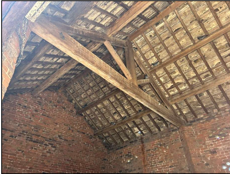
Photograph 2- Timber roof trusses spanning between the front and rear elevation
