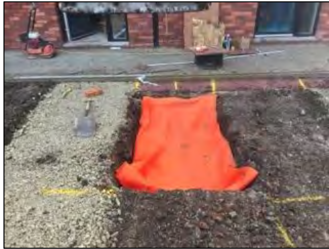
Figure 1: First, the gardens are dug out to 600mm below FFL and lined with a hi-viz geotextile marker:
