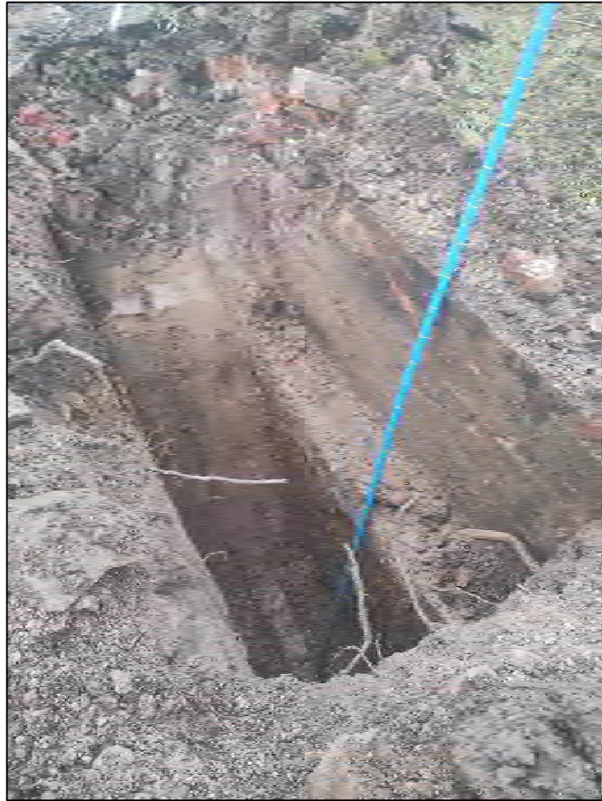
Figure 5: Footing feature encountered in TP101 in the footprint of the former boundary hotel.
