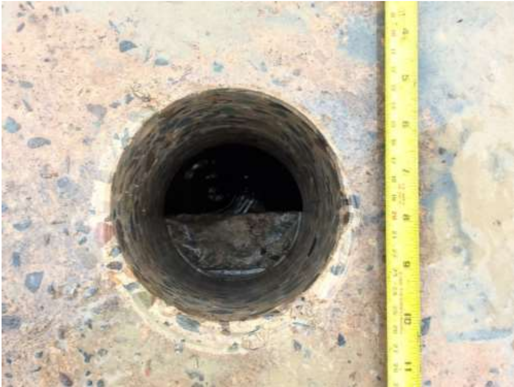
Photograph 9 View of T4 located within the tank.
