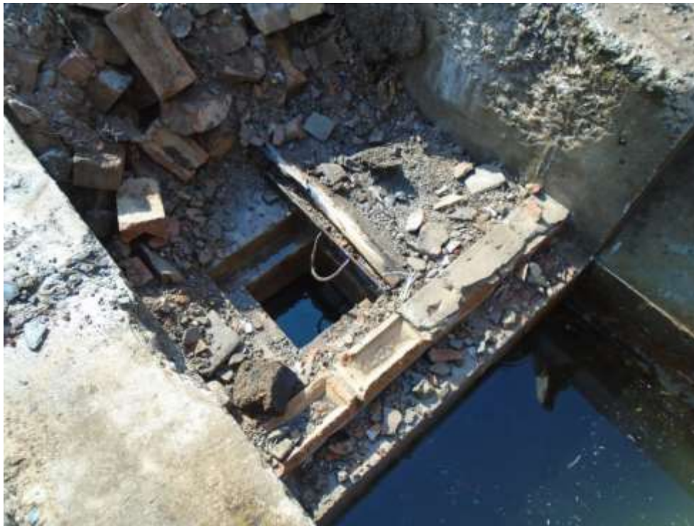
Photograph 3 View of the eastern side of the sump.
