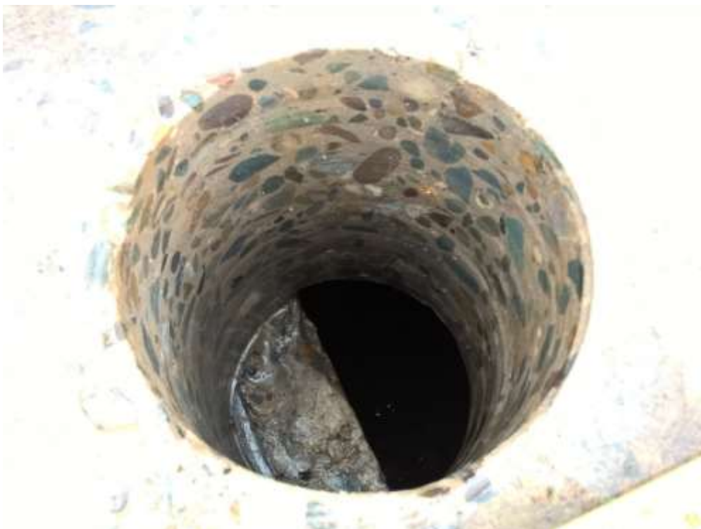
Photograph 10 View of T4 located within the tank.
