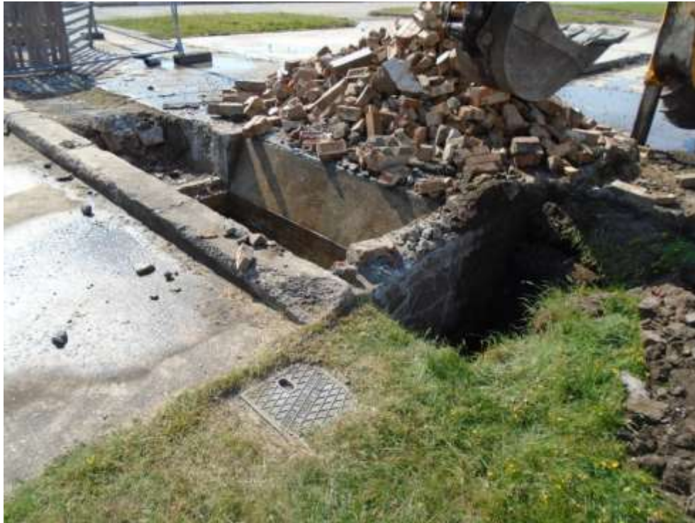
Photograph 5 View south-west towards the sump with the borehole in the foreground.
