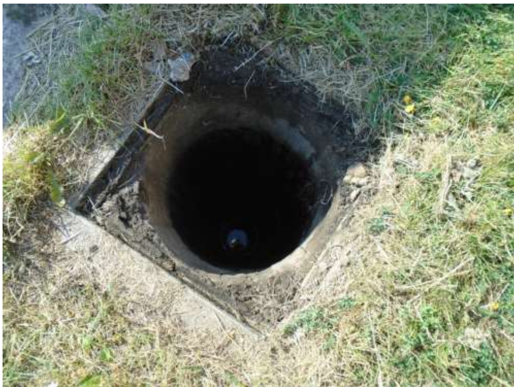
Photograph 4 View of the borehole adjacent to the sump.
