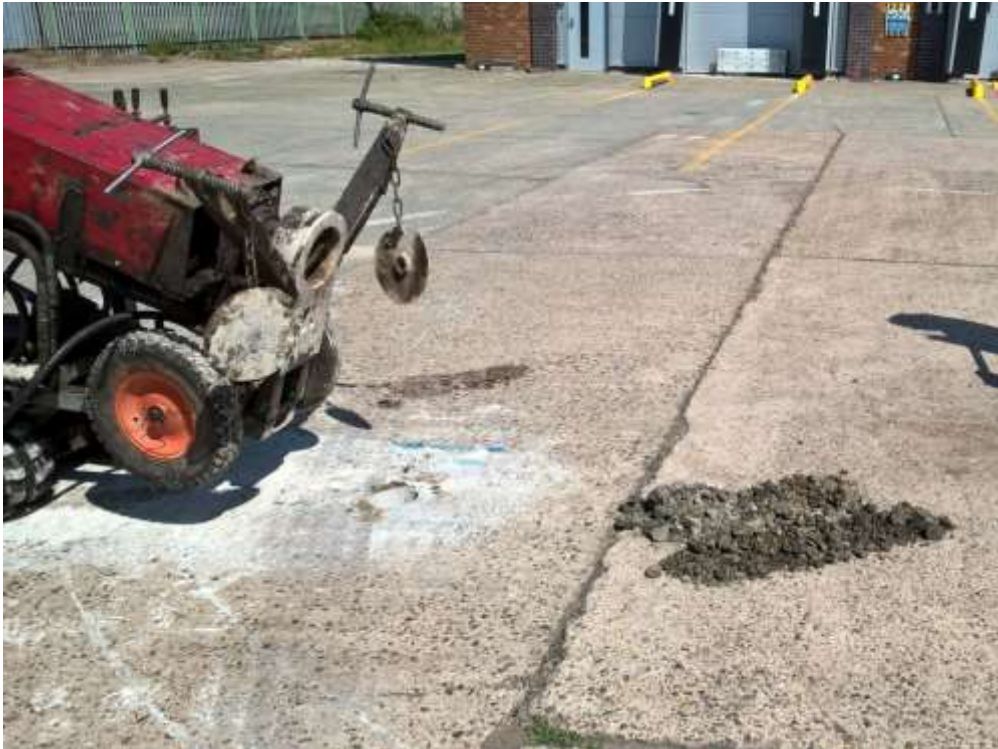
Photograph 7 View east showing the location of T3 north of the tank.
