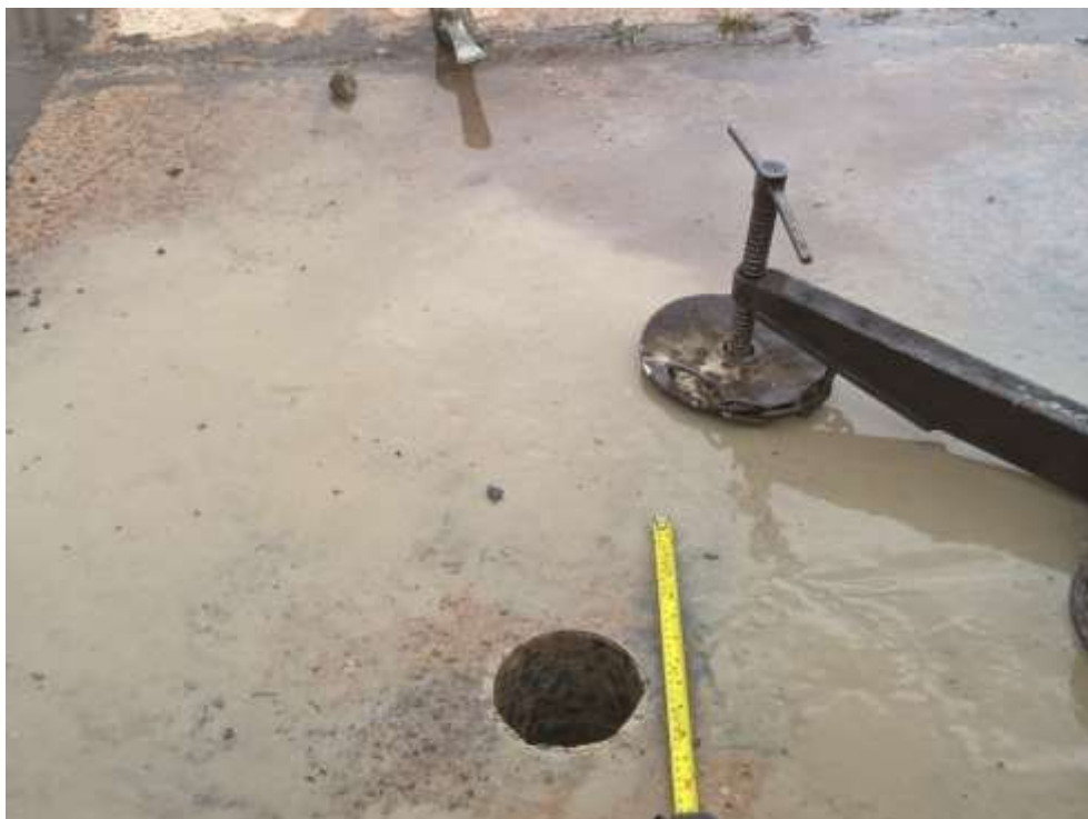
Photograph 8 View south showing the location of T4 within the tank.
