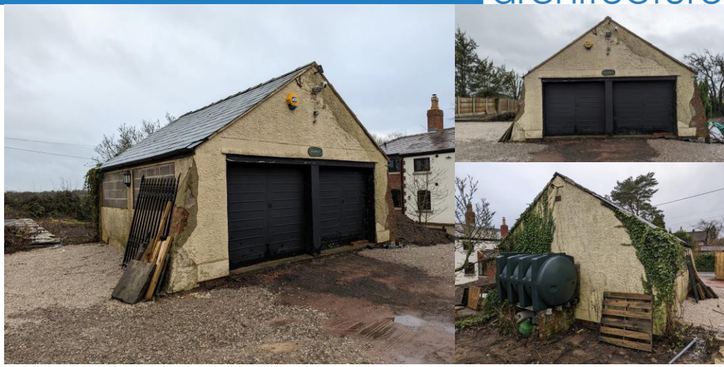
Figure 3.1 – Existing Garage to be Demolished
