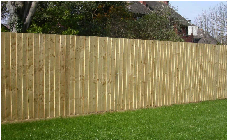
Close Boarded Timber Fence
