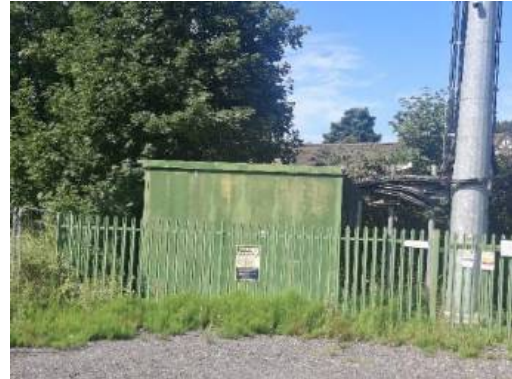
Photograph 2: Substation building (B1) located in western section of the site.
