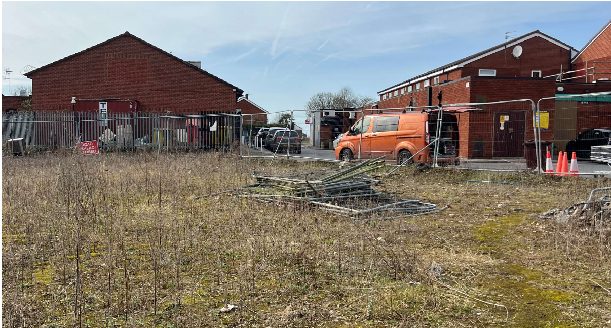
Figure 5 – Image showing tidy nature of site, with security fencing being erected to deter unauthorised access
