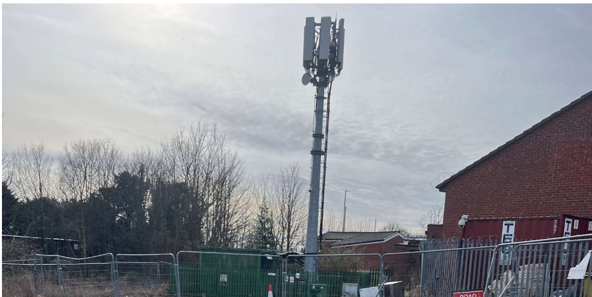
Figure 4 – Image of the telecommunications mast on site
