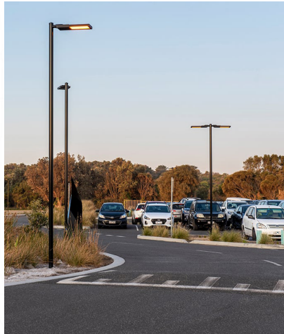
Column lighting for car park
