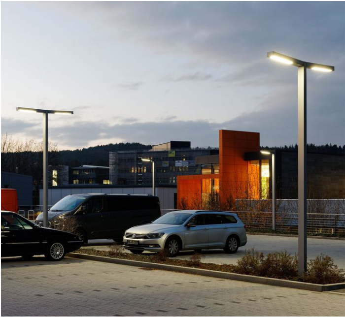
Utilising multi-head lighting columns for car park
