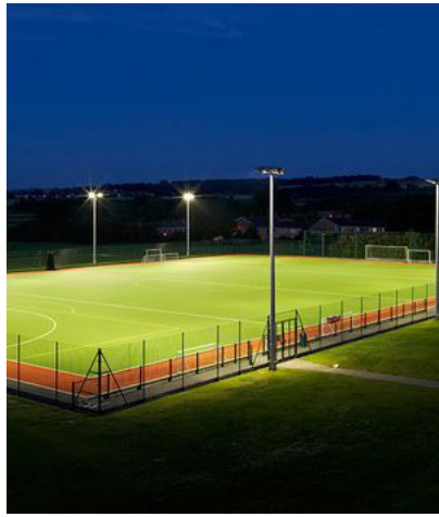
Floodlighting at football pitches
