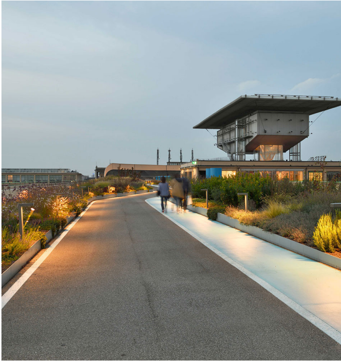
Low level lighting to active loop
