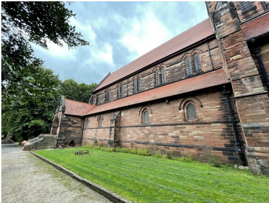
Figure 4.3: The south aisle of the Church of St Chad
