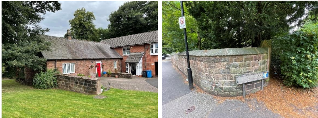
Figure 4.6: Views of the Stables and Gate Piers
