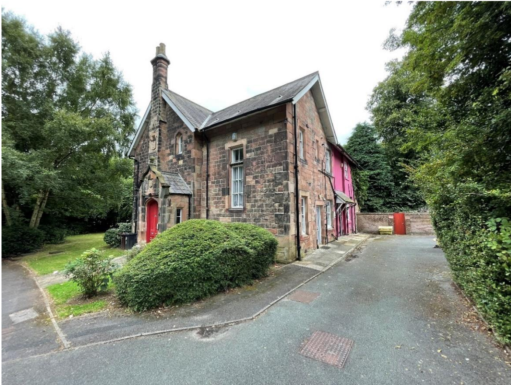
Figure 4.5: View of the Vicarage
