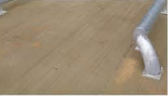
Concrete to yard areas and building circulation footpaths
