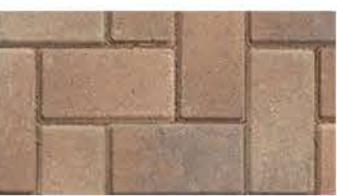
Block paving to footpaths
