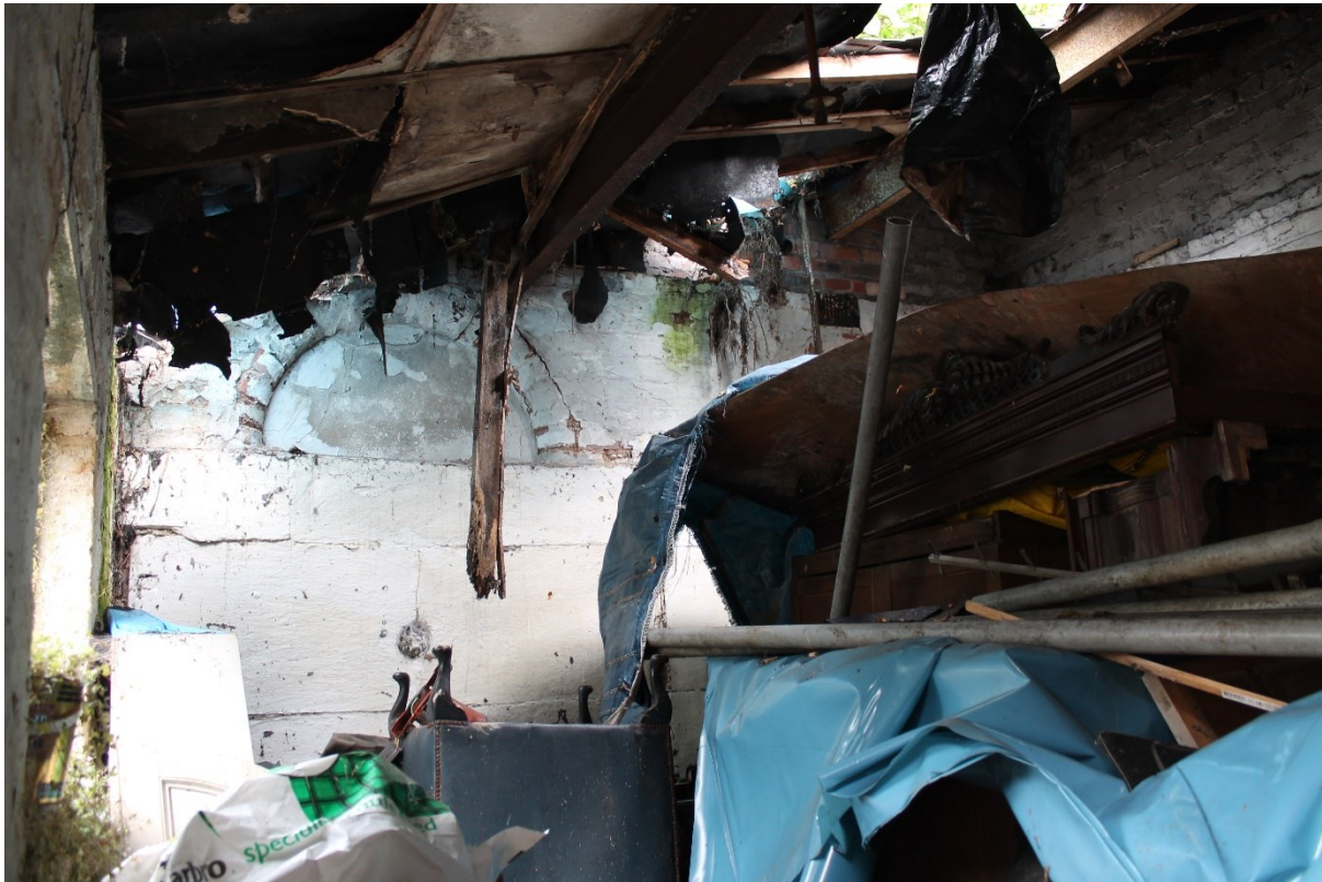
Figure 5.6: Interior of west bay
