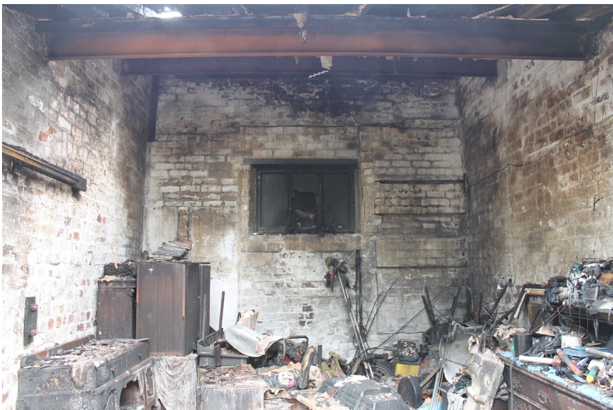
Figure 5.5: Interior of middle bay (note change in rear wall, steel beams and modern window)
