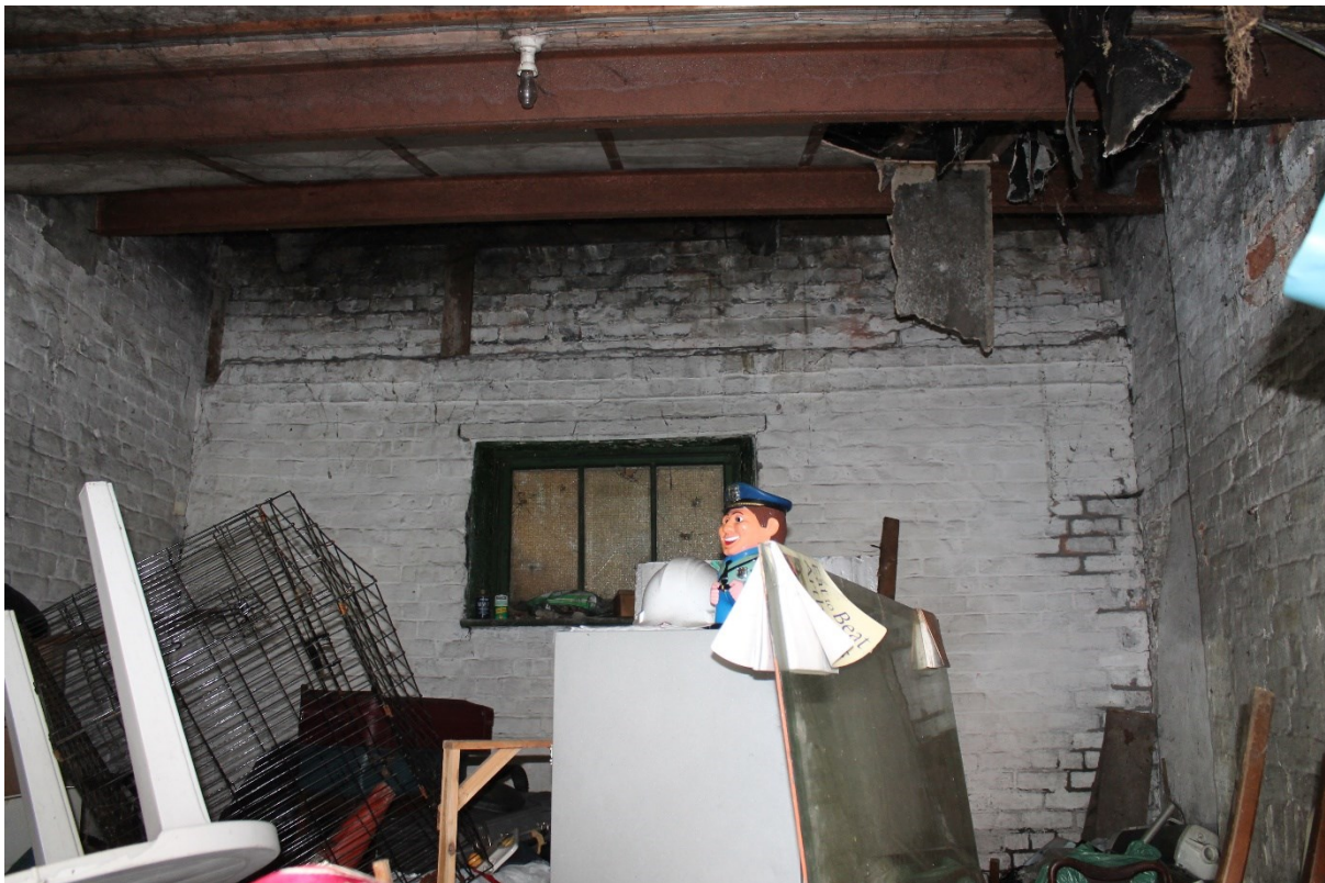
Figure 5.7: Interior of eastern bay
