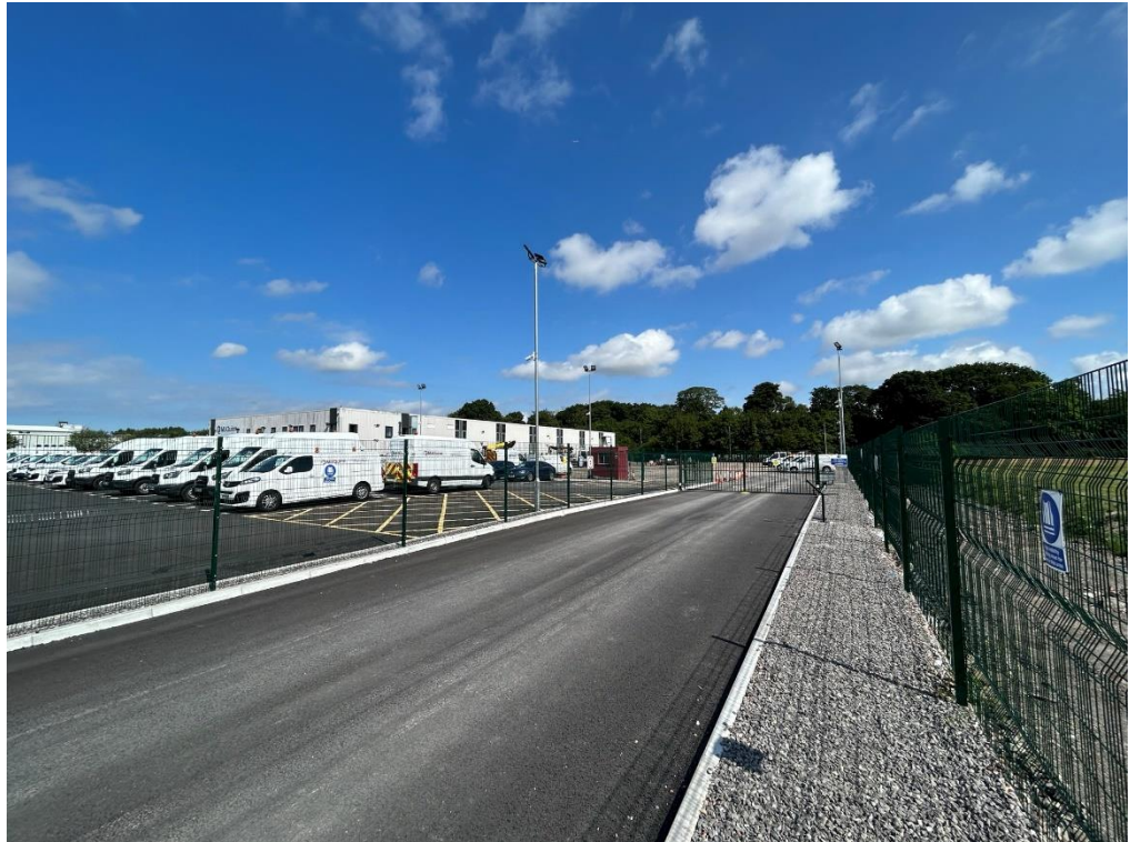
02 – Entrance road off Randles Road looking into the site.
