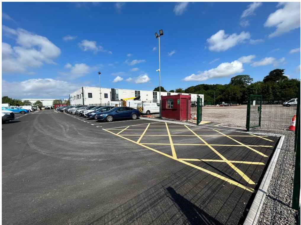
03 – Car park lighting.
