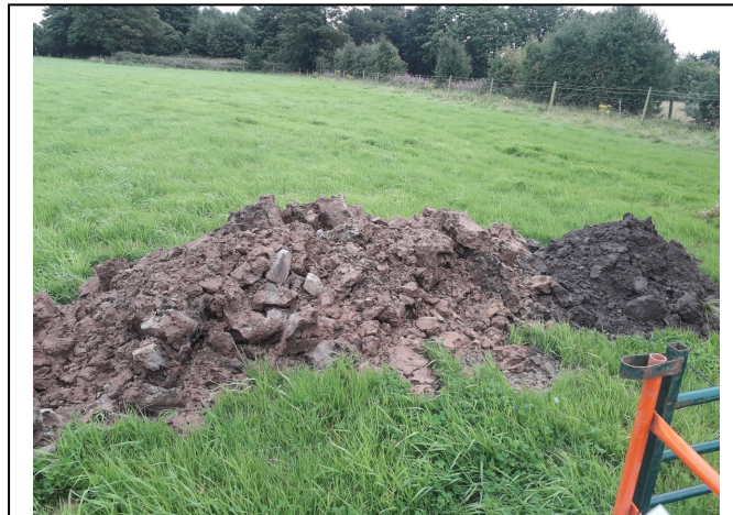
Trial Pit 106/ Soakaway 104 Spoil
