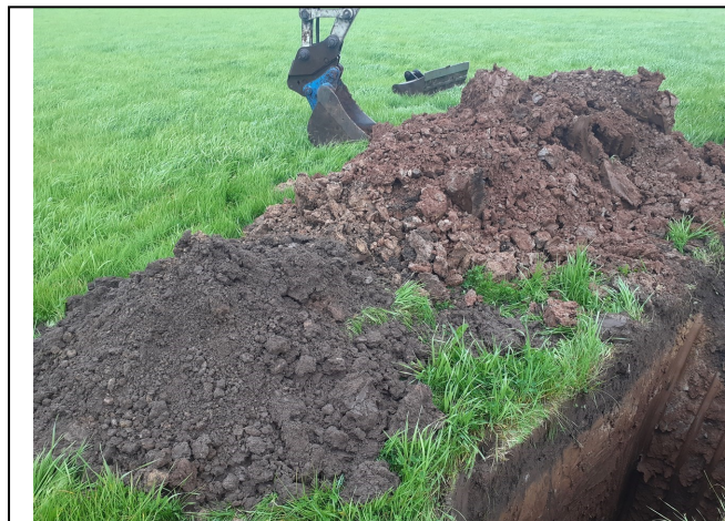
Trial Pit 120 Spoil
