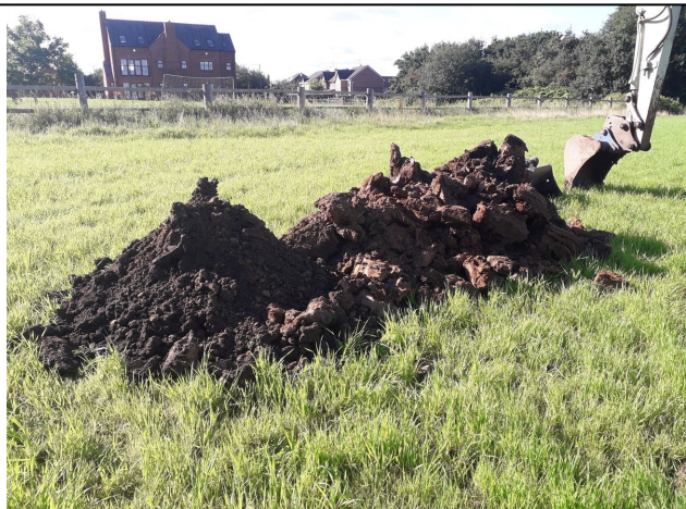
Trial Pit 101/ Soakaway 101 Spoil
