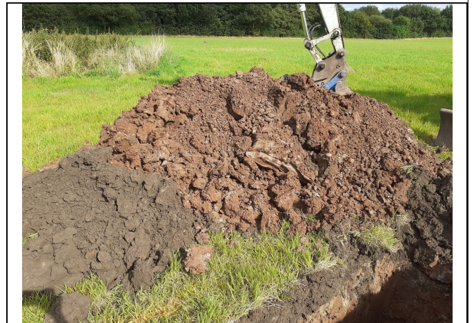
Trial Pit 118 Spoil
