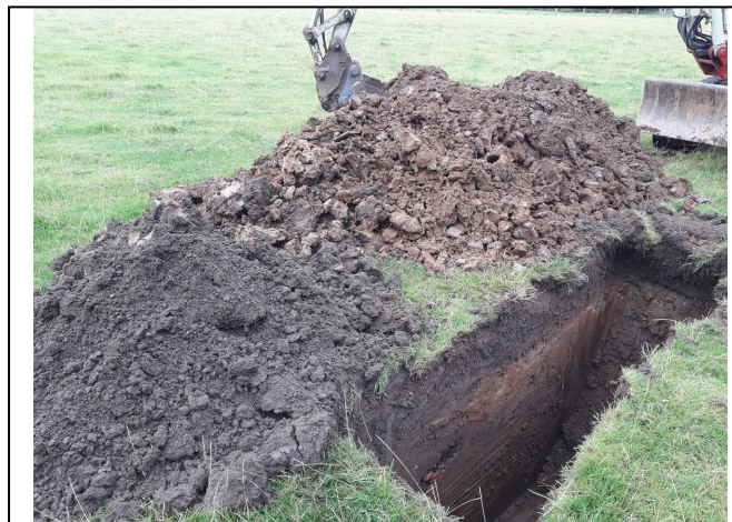
Trial Pit 136 Spoil
