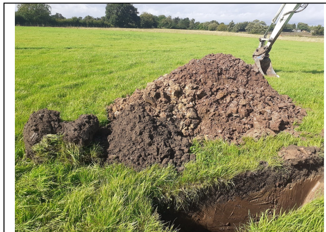
Trial Pit 125 Spoil
